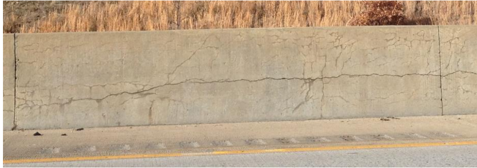
Figure 2.2. A typical median barrier section which exhibits moderate damage, (e.g. moderate visible map cracking, and a longitudinal crack along the full length of the section). Picture used with permission from Richard Deschenes.
