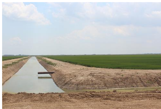
Figure 1.2: Tail-water recovery ditch collects water from fields ( Fritscher, 2015 )
