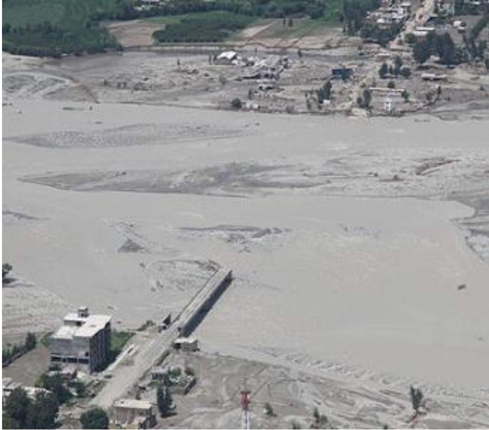
Figure 2.4: an example of a damaged bridge - Pakistan flood-2010 (adapted from EPACHA, 2010).
