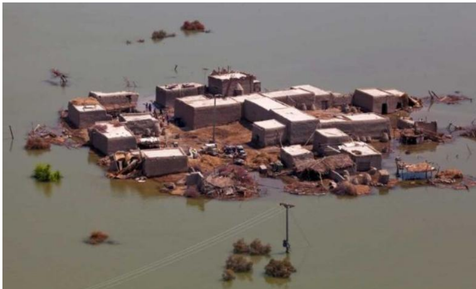
Figure 2.5: An example of houses surrounded by floods - Pakistan flood, 2010. (Adapted from: www. stamfordadvocate.com ).
