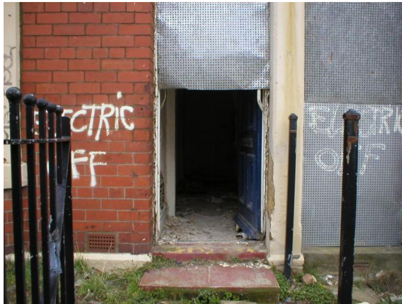
Figure 7.8: Signs of disconnection before demolition (Andrea Armstrong)
