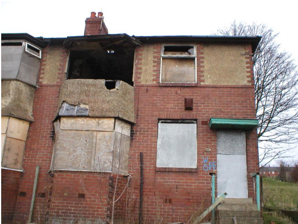
Figure 7.4: Tyneside flat in Scotswood awaiting demolition (Andrea Armstrong)
