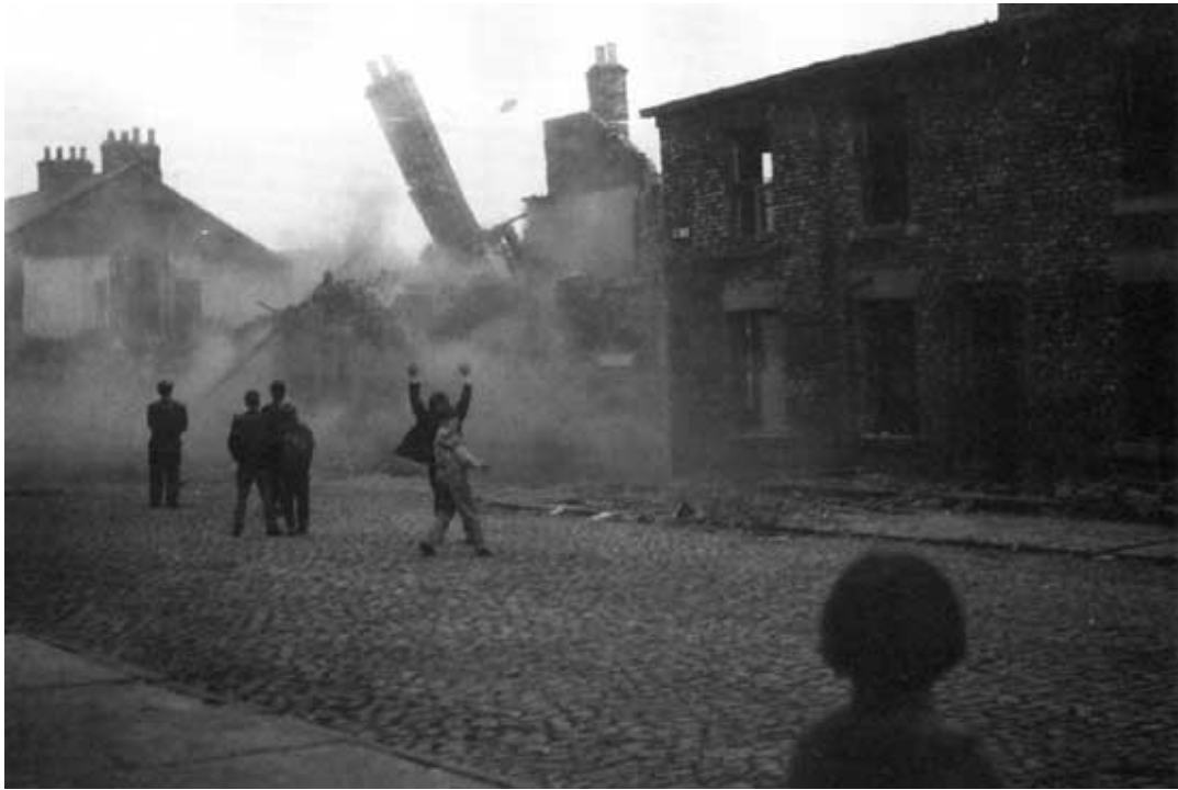
Figure 7.1 Demolition in Newcastle, 1960 17
