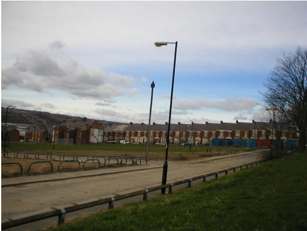
Figure 7.2 Scotswood after demolition in 2007 (Andrea Armstrong)
