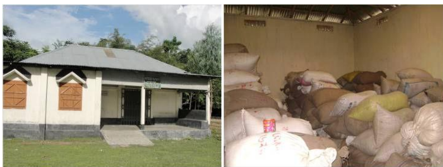
Photograph 7.2: The left photo shows the Community Dhan Bank and the right photo shows the paddy stock in the Dhan Bank godown (warehouse).
