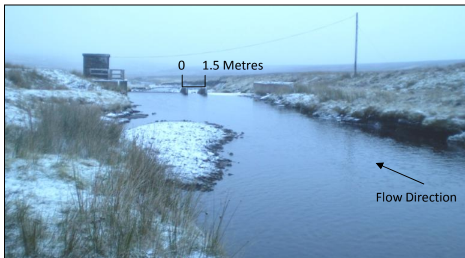
Figure 3.1 EA compound weir gauging station on Trout Beck, downstream of the study reach.
