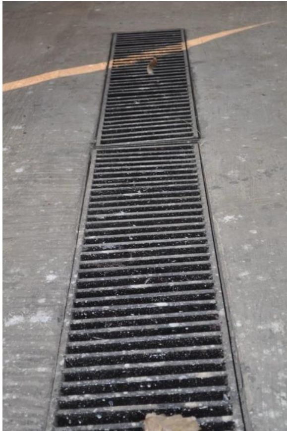
Figure 6.4: Simple storm drain collection designed to exclude leaves (Source: Author)
