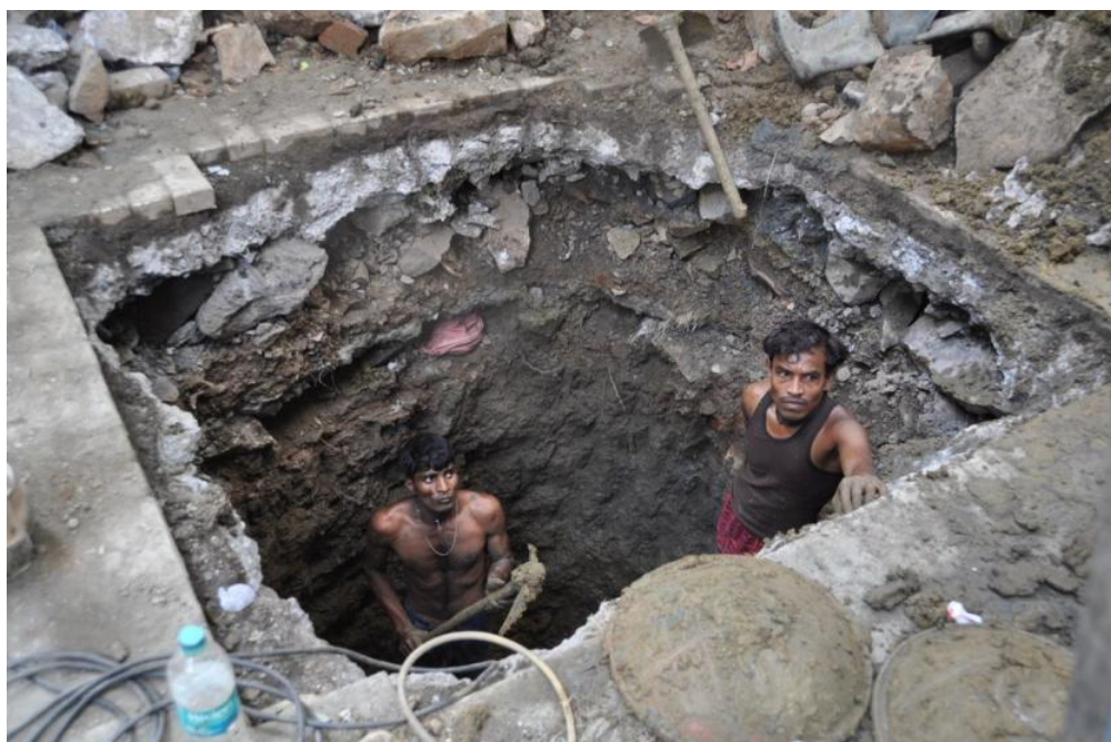
Figure 6.8: The well is dug by hand (Source: Author)
