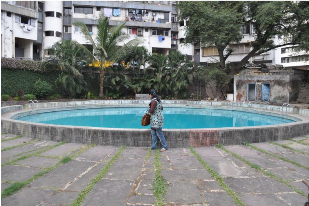
Figure 7.4: Rarely used swimming pool filled with harvested rainwater, Kanti Apartments, Mumbai (Source: Author)
