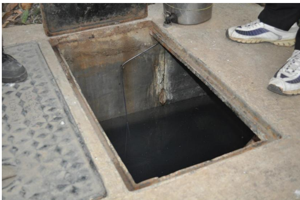
Figure 6.11: Chemicals are added to this system everyday (Source: Author)
