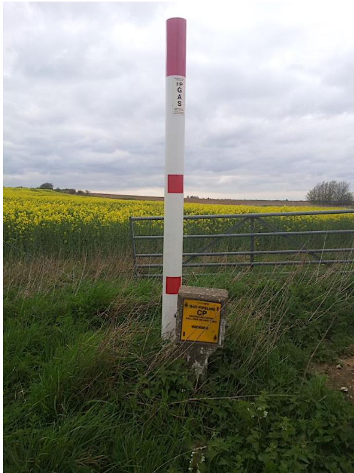
Figure 17 - Photograph of NTS pipeline marker in Norfolk, 2014
