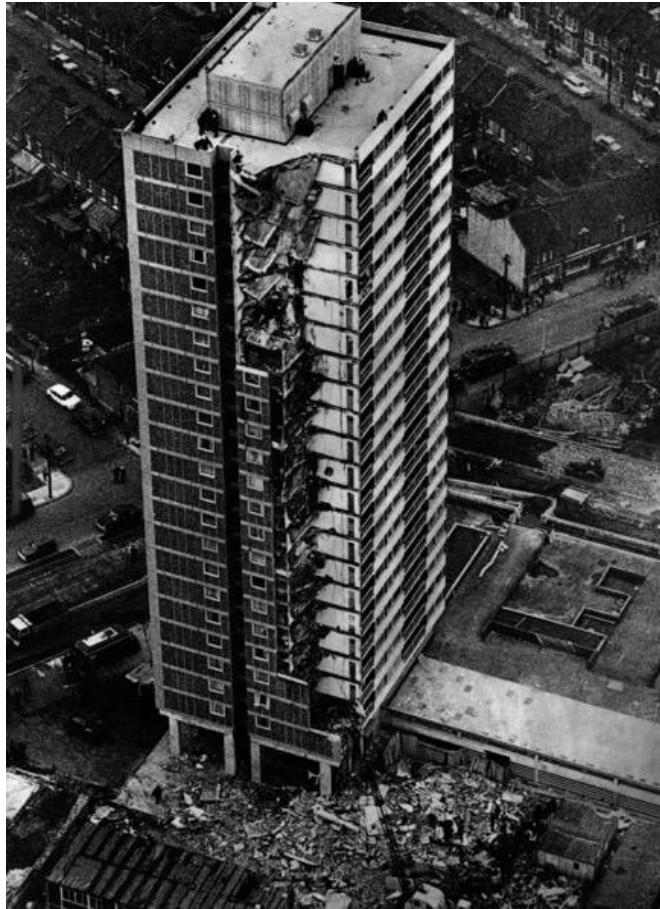
Figure 11 - Photograph of Ronan Point, 1968
