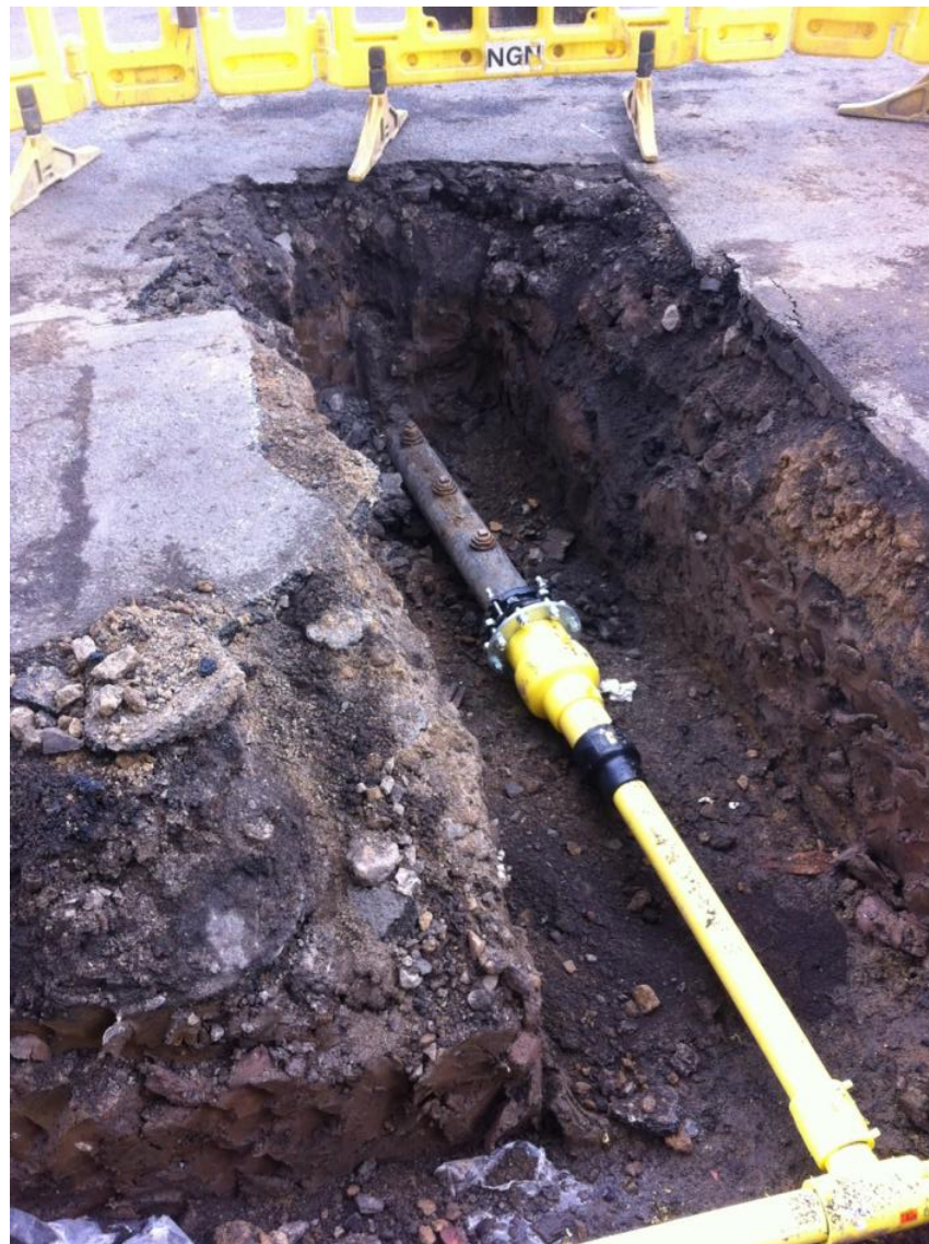
Figure 18 - Photograph of a distribution pipe in Middlesbrough, 2015
