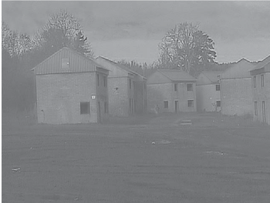
Fig. 4.87.: The result of applying the High-Pass Regional Variance method to the images in Figure 4.10
