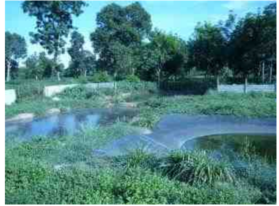
Photo 4. Ponding system. Upon removal of solid waste from the piggery floor, wastewater might be treated in a ponding system. These systems can be sophisticated and in the case shown it includes a covered subsurface flow constructed wetland (notice the rubber leaning with water accumulation on the top) and a second and third polishing pond (right upper corner), Yasothon Province, August, 2008.
