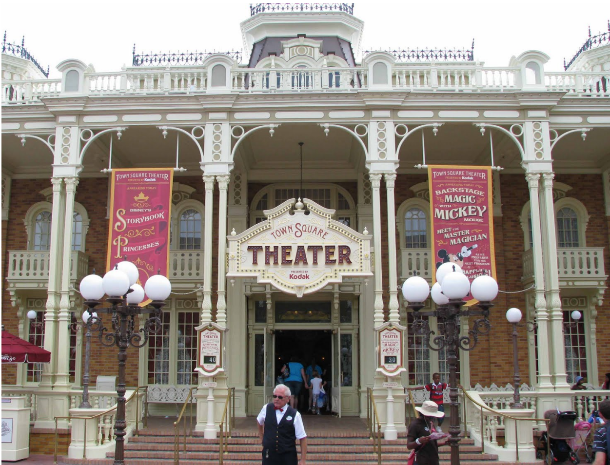
Figure 6. Architectural details of Town Square Theater (Author's Photograph, 2013).
