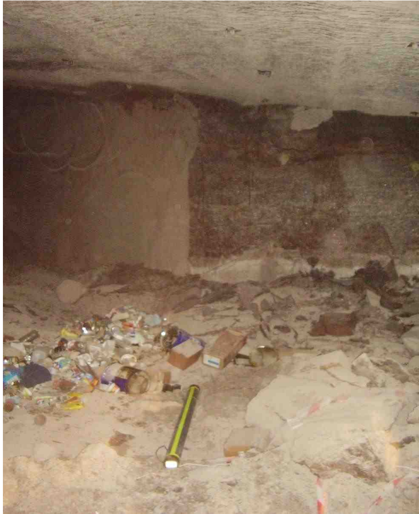
Plate 5.2 Closuremeter installed at cross-cut at site 2 in the North
