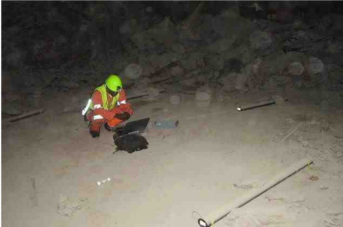
Plate 5.3 Closuremeters installed in parallel at stub at site 3 in the North
