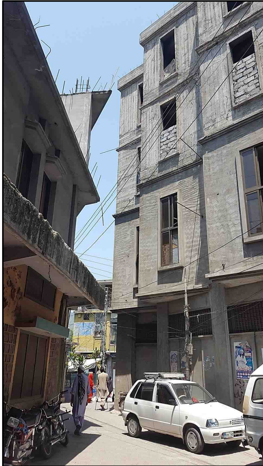
Figure 7.14: Newly constructed multi-storey buildings in the congested old city area of Muzaffarabad. Notice narrow street and addition of new storeys on an old dilapidated building on the left. (Source: Author fieldwork)
