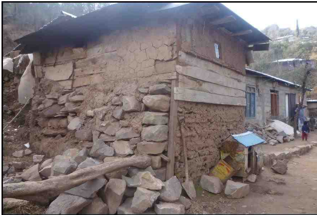
Figure 7.8 A poor quality structure (foreground) added with a reconstructed house (background) in Bagh city; notice different types of materials and irregular stones used in the added structure. (Source: Author fieldwork)
