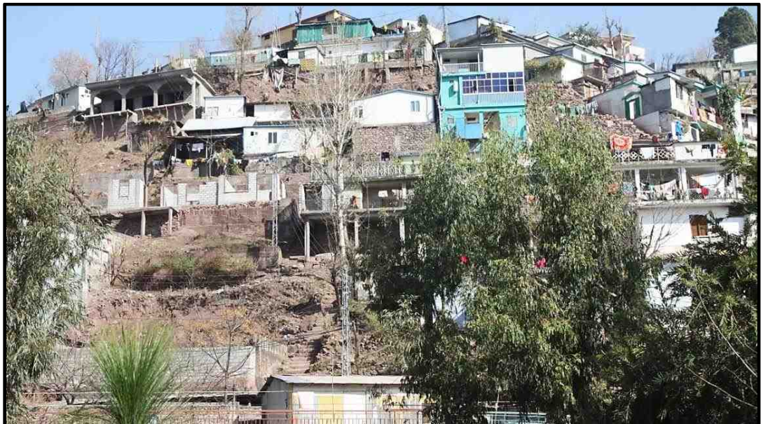
Figure 7.11 Construction on steep slopes in Muzaffarabad city; these houses have been built by cutting the hill. Almost half the house is on ground and half of stone pedestal or concrete pillars which seriously compromises the safety of the structure.
