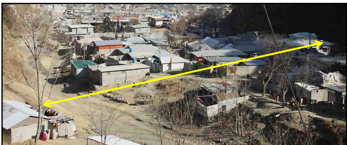
Figure 7.13 Construction in the Gojra Nullah; the yellow arrow shows the width of the nullah that has been taken over by illegal houses. (Source: Author fieldwork)
