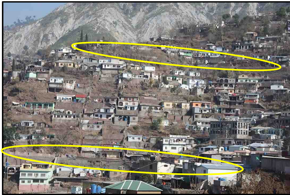
Figure 5.18 Massive building and road construction (yellow circles) on steep slopes in Muzaffarabad city. All the construction has been done after doing earth cutting.
