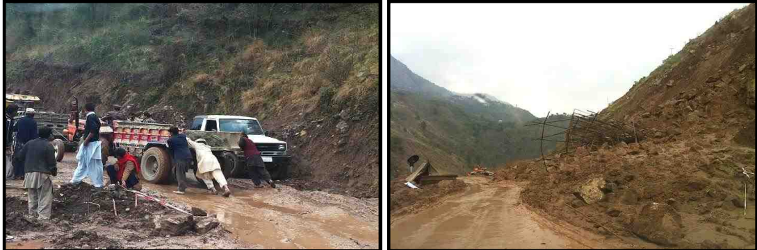
Figure 9.2 Landslide hazard on the roads.
