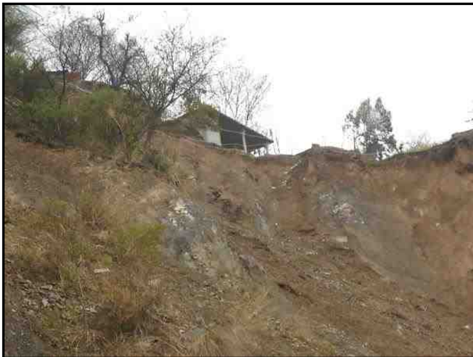
Figure 7.17 A house facing immediate collapse due to landslide in Lohar Gali area of Muzaffarabad District. (Source: Author fieldwork)
