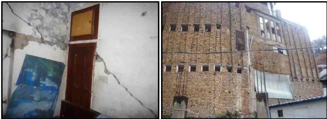
Figure 7.7 A damaged house in Bagh city which has been partially repaired and still inhabited by the owner and his family (left). A pre-earthquake multi storey commercial building in Bagh city, non-frame structure and cracked walls pose serious threat (right). (Source: Author fieldwork)
