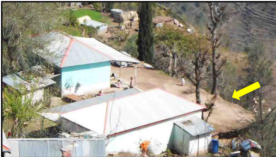
Figure 5.3 A Pukka house in rural area with a kacha cattle shed or gohaal (yellow arrow) added with the house which serves as courtyard as well; notice shear fall in front of the cattle shed. (Source: Author fieldwork)
