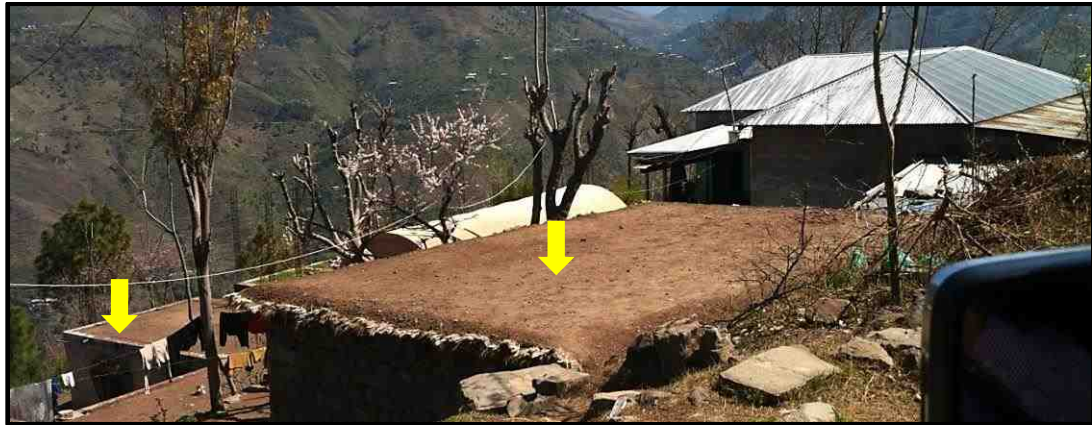
Figure 7.9 Kutcha structures (yellow arrows) added with reconstructed pukka house in rural Muzaffarabad. (Source: Author fieldwork)
