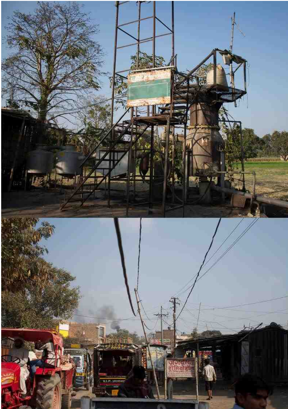
Figure 5-5: Locally fabricated gasifiers and transmission lines on bamboo sticks.
