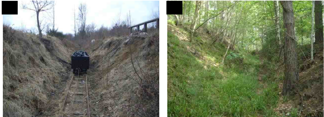
Figure 5.6 (A) Winter photograph of the western coal tubway cross-section from the position of transect B in figure 5.12. Note the tubs and tracks are replicas placed at this site for heritage value. (B) Summer photograph up the southeast tubway from the position of transect B in figure 5.7, with pine forest cover.
