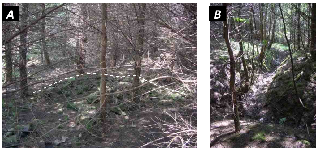
Figure 5.27 (A) Winter photograph of one of the building rubble piles at test site 8 with the shape of the pile highlighted. (B) Winter photograph from the northern end of the man-made channel at test site 8 (note the fork). Both features lie under Douglas fir canopy.
