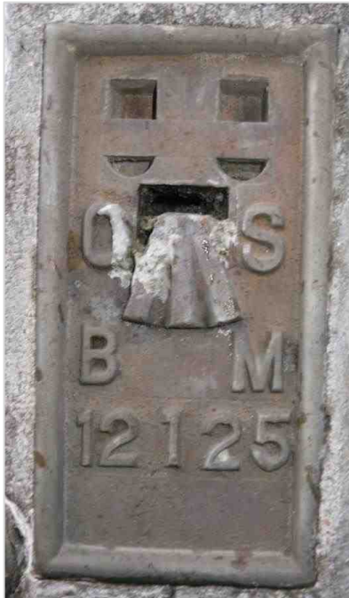
Figure 4.1: Flush bracket 12125 at Clashnessie Bridge, located at 10.343 m OD, used to relate the survey data from each site to the national levelling datum for the UK, Ordnance Datum (Newlyn).
