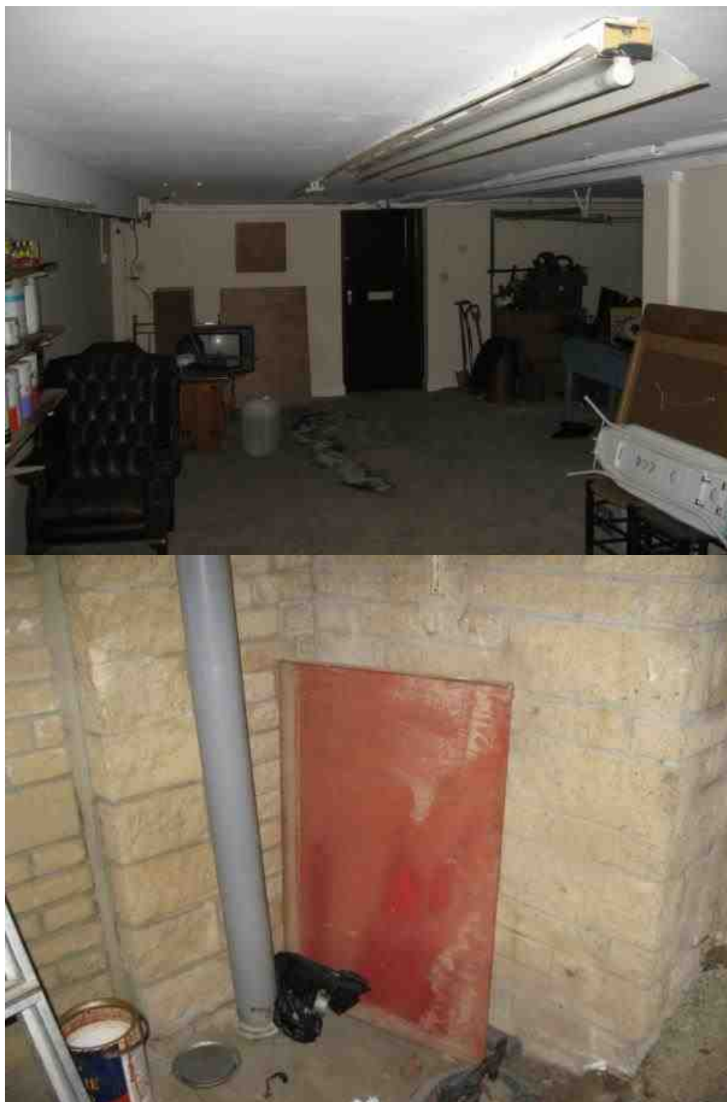
Figure 5.3: Two adaptations to flooding at a house in Helmsley. Top: the lower floor of the house, not used as a living space and largely cleared out of valuables. Bottom: a wooden barricade.
