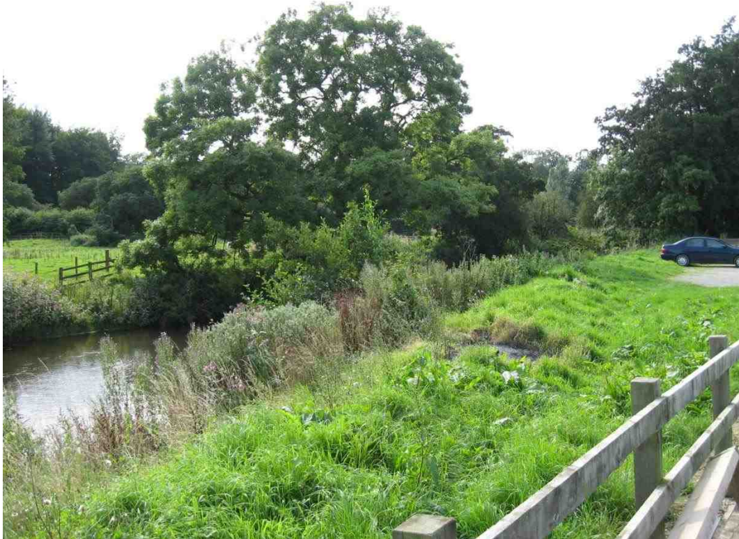
Figure 5.4: The raised river bank of the River Rye, work completed prior to the 2005 flash flood, built between the River Rye and the houses in Bridge Farm Close and Ryegate in Helmsley.
