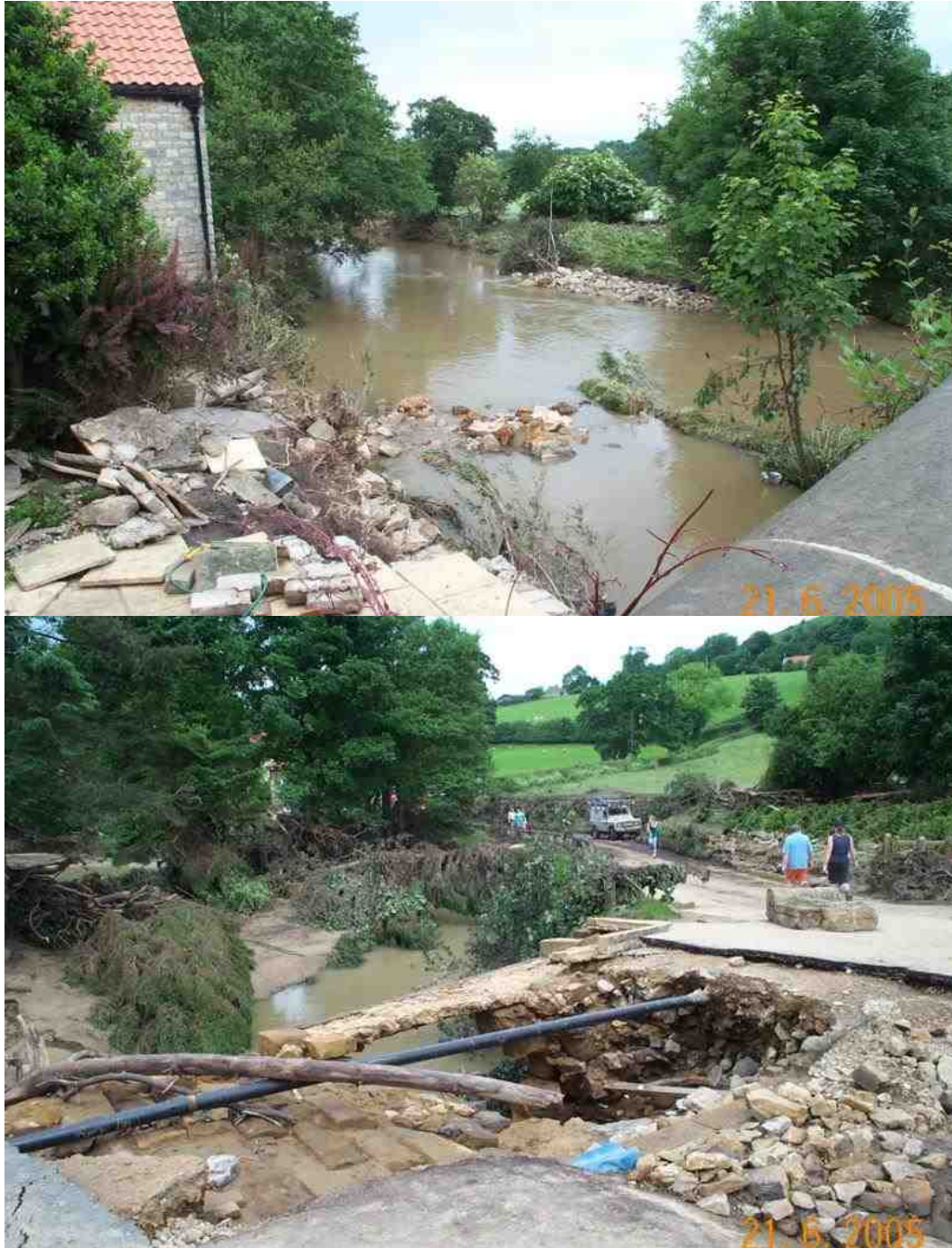
Figure 1.5: Damage caused by the 2005 flash flood event in upper Ryedale, photographs taken at Helmsley (top) and Hawnby (bottom), showing damage to infrastructure and property in addition to the deposition of large amounts of fine sediment and debris. Photographs provided by Jeff Warburton.
