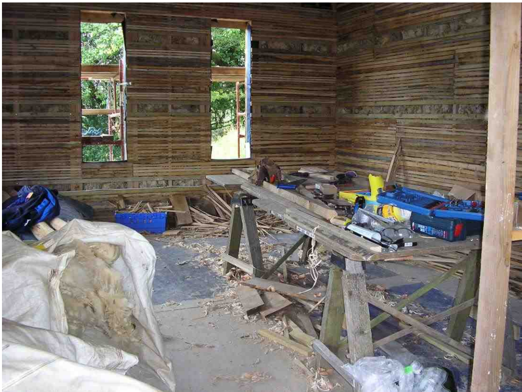
Figure 25: clutter of materials and tools inside the barn, (photograph: authors own)
