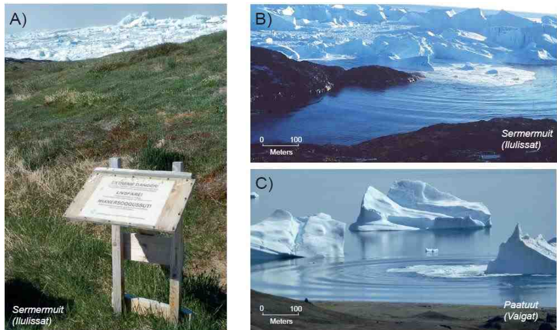
Figure 5.2. Iceberg tsunami hazard in Disko Bugt, west Greenland. (A) Public warning notice of the threat of iceberg-generated tsunamis, posted by the Ilulissat Municipality. Sign reads “EXTREME DANGER! Do not walk on the beach. Death or serious injury might occur. Risk of sudden tsunami waves, caused by calving icebergs”. (B) Example of small iceberg-generated waves from Ilulissat (close to site of A, credit Dr David Roberts) and from near to Paatuut (C).
