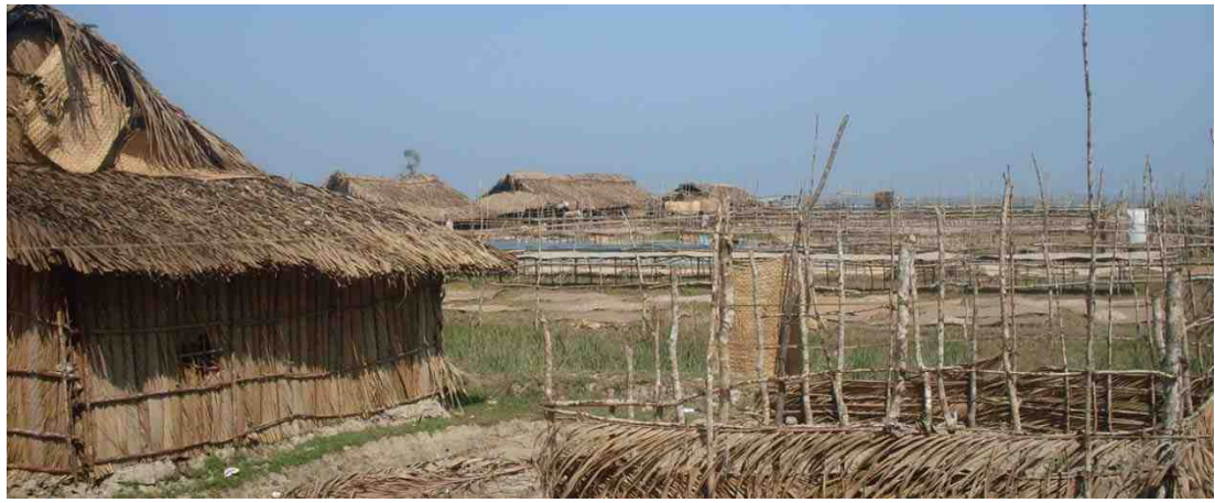
Figure 8.7: A temporary fishing village (inhabited from September – April fishing season) in a Sundarbans Island, called Shewlar Char . Houses are made of nol , son and golpata . (Source: Author, 30/01/2010)
