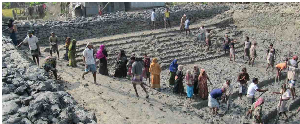
Figure 3.2: A Water Tank Digging Work under a 'Cash for Work' Project, where Men and Women are Working Together (Source: Author, 10/11/2009).
