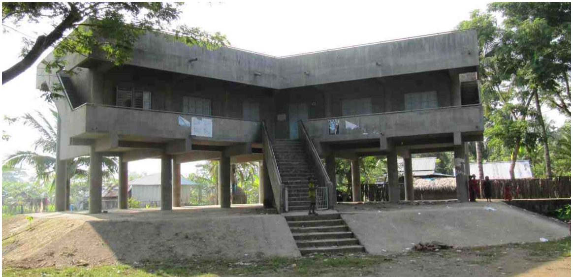
Figure 4.4: Gabtola Cyclone Shelter
