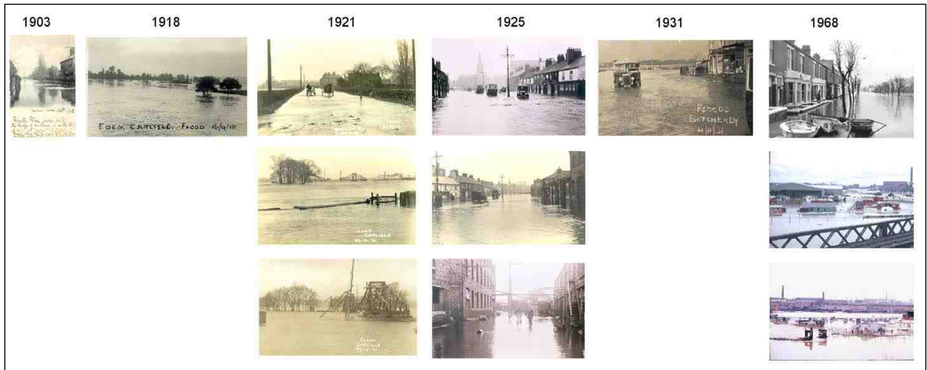
Figure 4.6 Photographs of flooding in Carlisle over the past 100 years.
