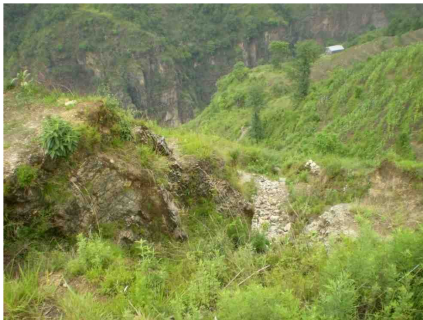
Figure 4.20 Terraces destroyed by the active translational slide at the bottom of Marmin settlement.
