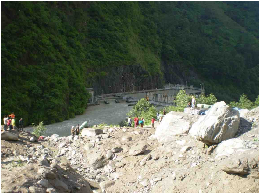
Figure 4.17 The Tatopani debris flow reactivated following heavy monsoon rains in July 2007. Landslide material partially blocks the Bhote Koshi River behind the Tatopani hydropower dam.
