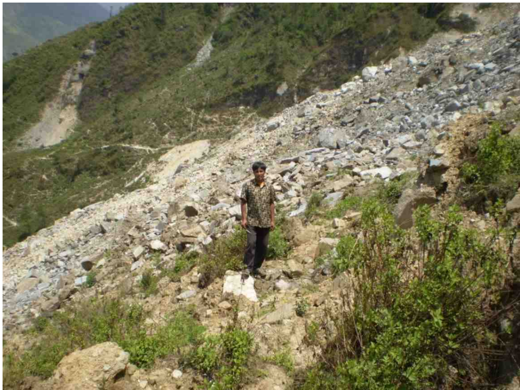
Figure 4.23 The 2006 Chambang landslide.
