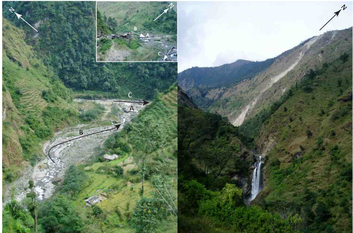
Figure 4.15 Left - The Bhairab Kunda Khola. Extensive aggradation and erosion caused by the 1996 channelised debris flow resulted in the loss of farmland and the lateral migration of the stream channel. The Bhairab Kunda Khola (B) joining the Bhote Koshi River (C) below Larcha bridge (A). The inset shows the settlement of Larcha at the confluence of the Bhairab Kunda Stream and the Bhote Koshi River. Right – An active gully depositing material into the Bhairab Kunda Khola approximately 750 m upstream from Larcha.
