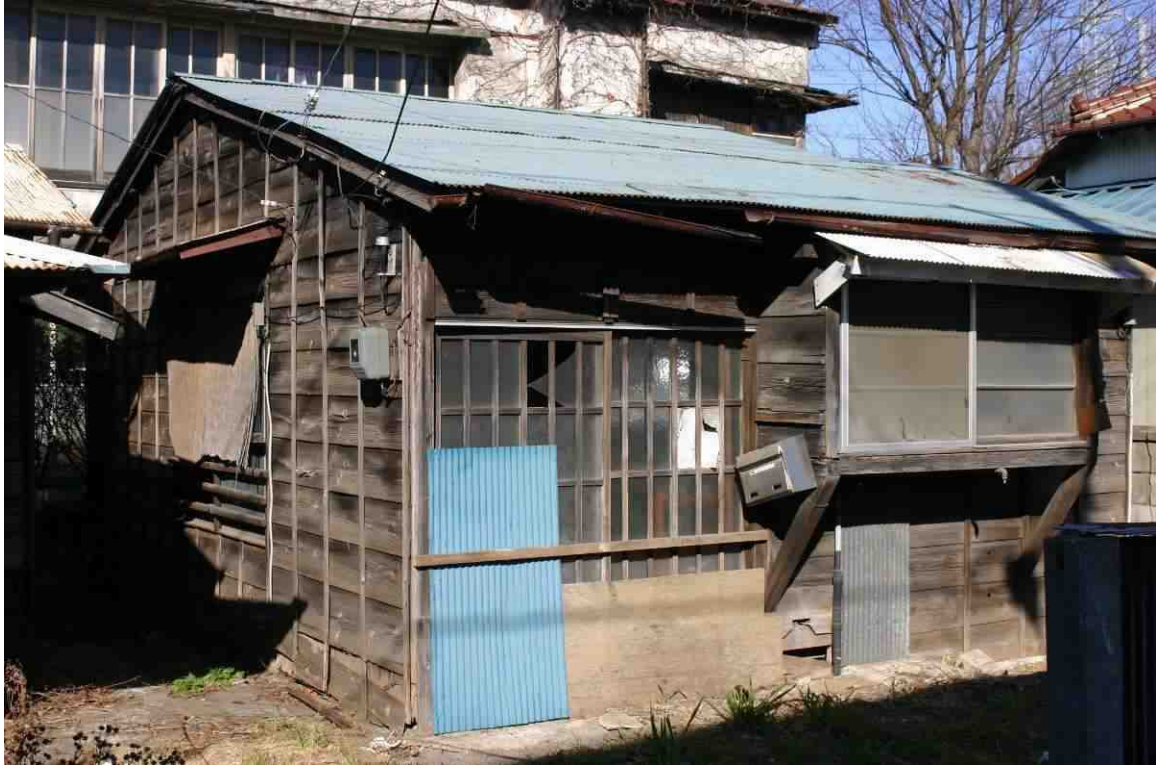
Fig. 6.8: Carpenter constructed house from about 1952. Before tin cladding was available for plywood cedar shingles continued to be used for exterior cladding. Shioda-chō
