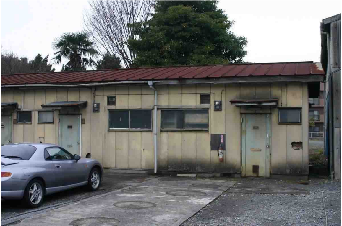
Fig. 7.12. One form of 'nagaya' tenement dwelling used for 'issued accommodation' by a joinery firm in Murata in the 1960's, now storage. It is very difficult to piece together any overview of this kind of dwelling at the period because it was almost all demolished by 1990.
