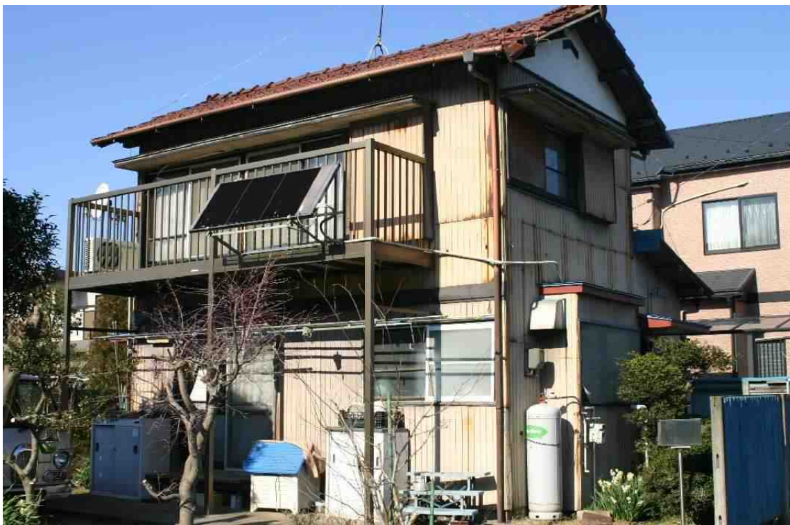
Fig. 7.14 Two storey dwelling design from the early 1960's. The use of zinc plated coating to protect the underlying plywood skin is typical of the period. No parking place. Benten 1-chome.
