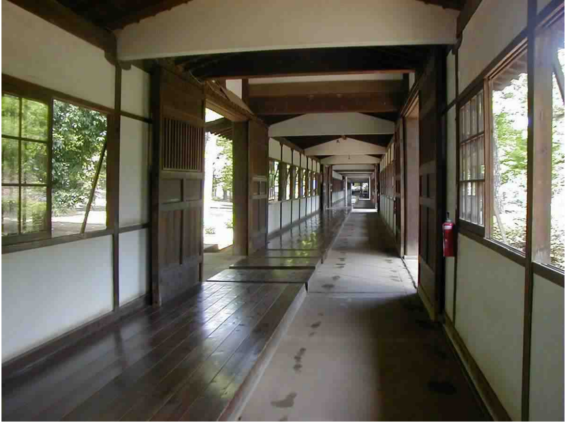
Fig. 4.8: Internal and external use combined. The raised highly polished wooden floor is for monks wearing slippers, the concrete for visitors in outdoor shoes. Sōjiji Temple, Tsurumi [IR]
