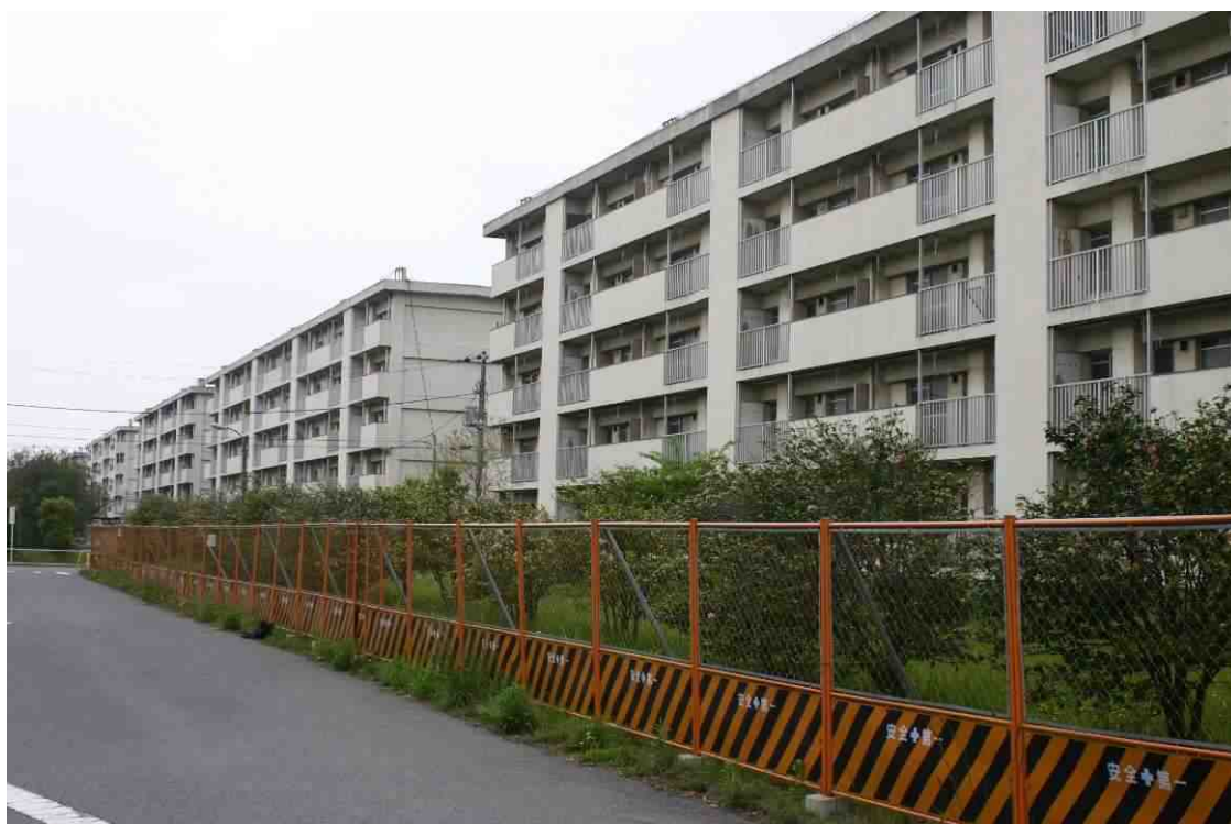
Fig 9.6: Some of the 730 late 1960's JHC apartment blocks vacated and sealed off ready for demolition and replacement by condominium clusters. Inage-kaigan 5-chome 2005. [IR]
