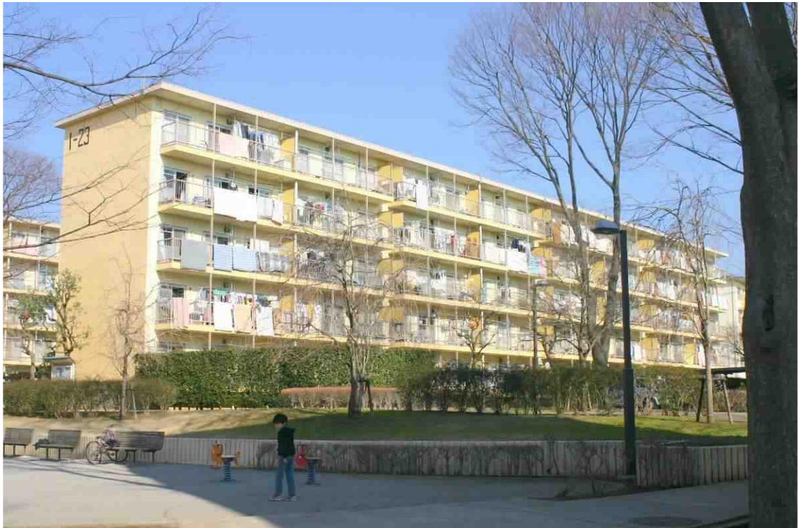
Fig 7.15. Four stairwell five storey JHUDC steel-framed ferro-concrete public apartment blocks completed in Hanamigawa-cho in 1967. There are over 90 similar blocks in this one danchi
