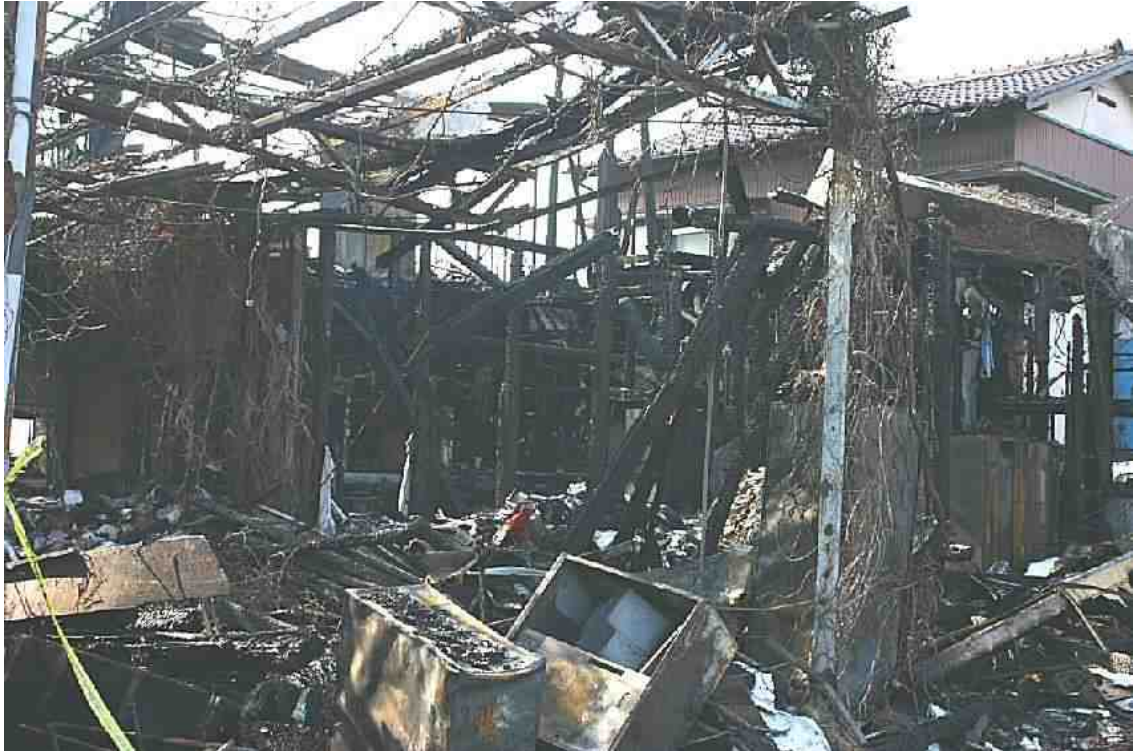
Fig.1.1. Even modern wooden framed dwellings are completely destroyed by fire within about twenty minutes. House fire at Nishi-Tsuga 4-chome January 2007
