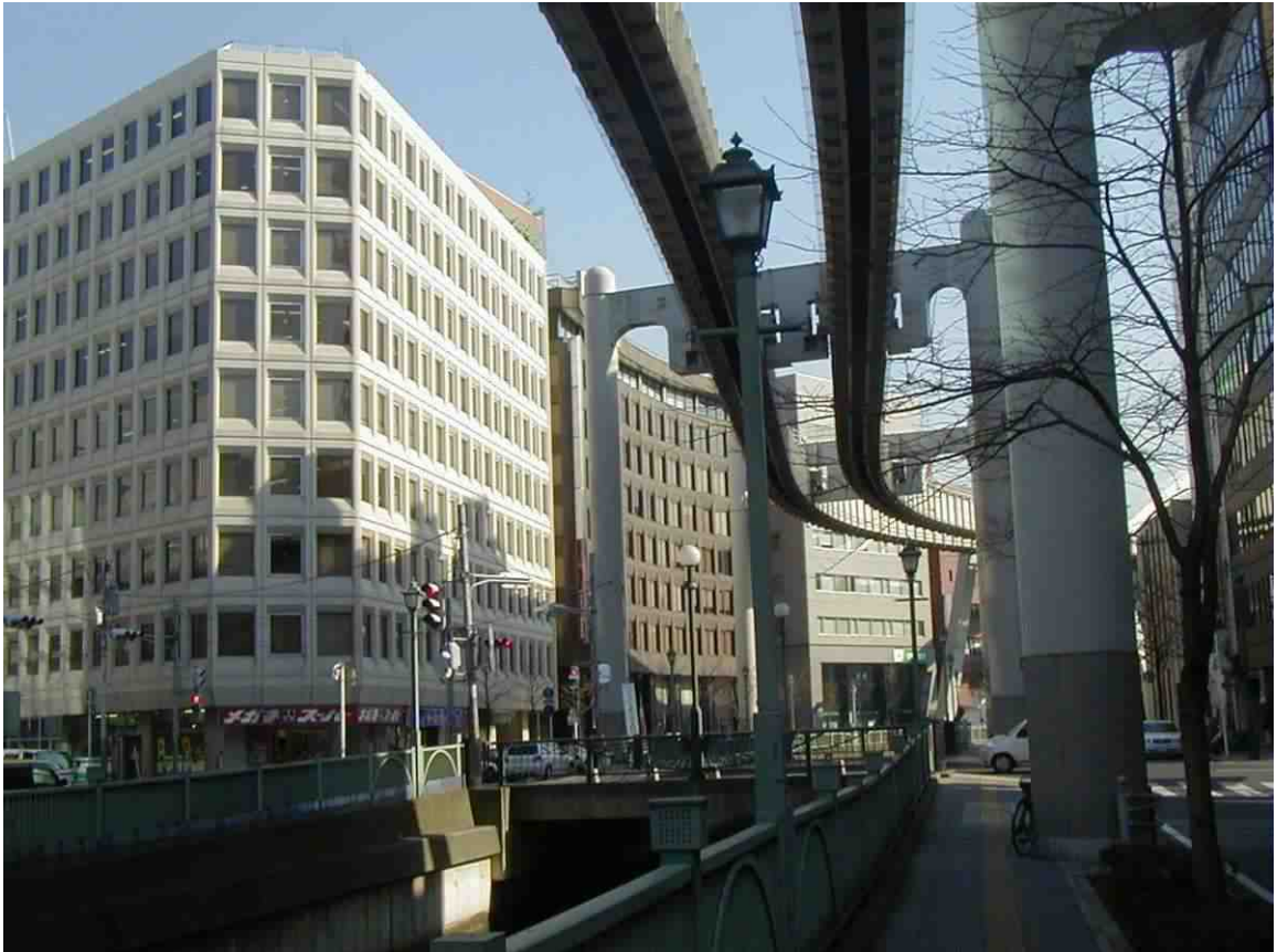
Fig. 6.5: Fujimi-chō was one of the few areas of Chiba to have 36m highways designated in a Sensai Fukkoin plan. The width proved useful later in the 1990s for the monorail project
