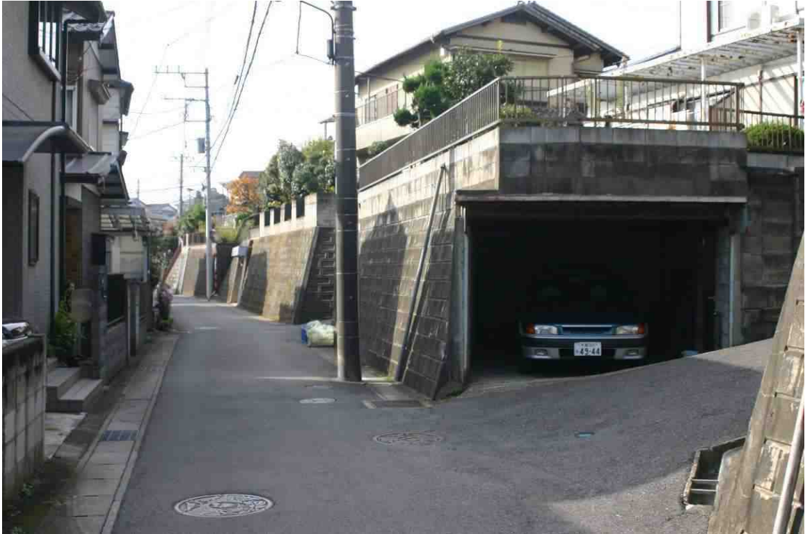
Fig. 4.3: Levelled building plots with concrete retaining walls from 1975. The slope here allows for garages under the garden, wooden houses above have living space facing south. Houses to left are similar but north facing kitchens and bathrooms face the lane access. Ō-mori chō [IR]
