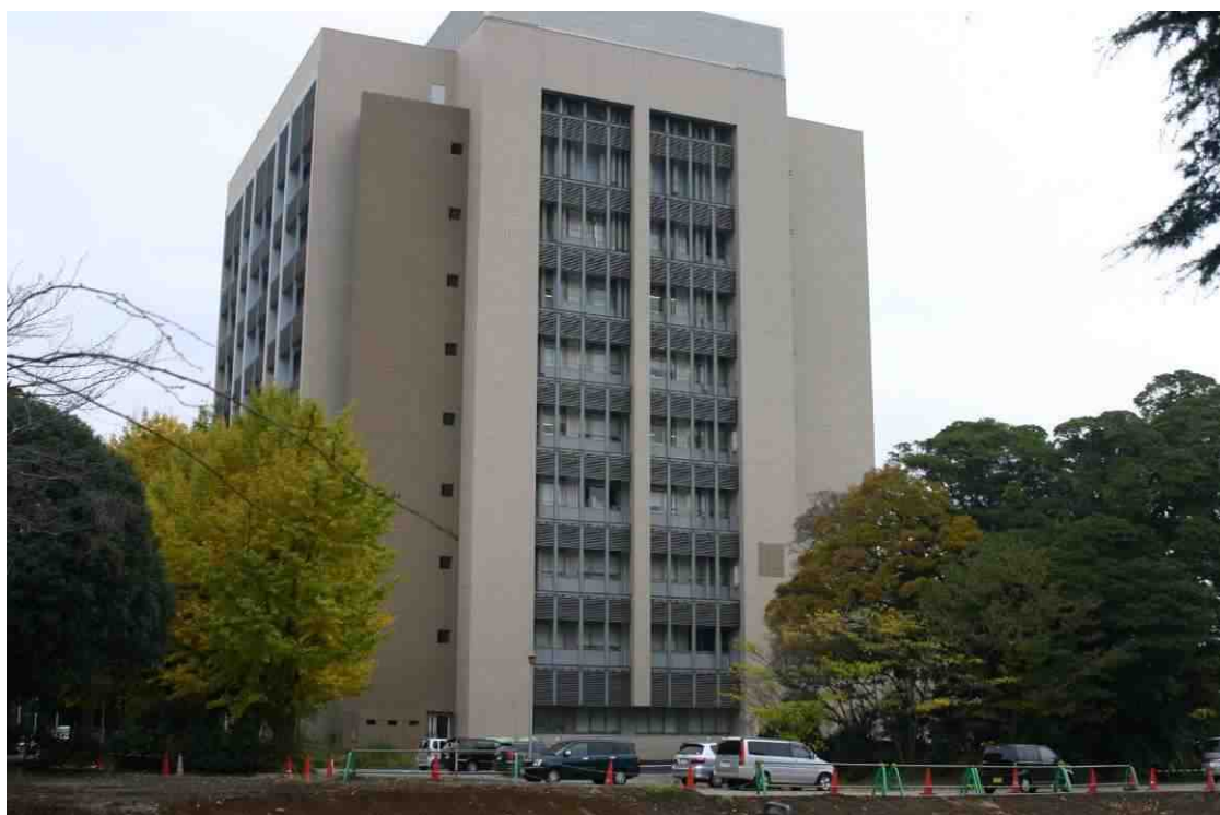
Fig. 9.5 Most of the growth in employment in this period came in service roles within larger establishments. One of four large extensions in the 1990's at Chiba University Hospital.
