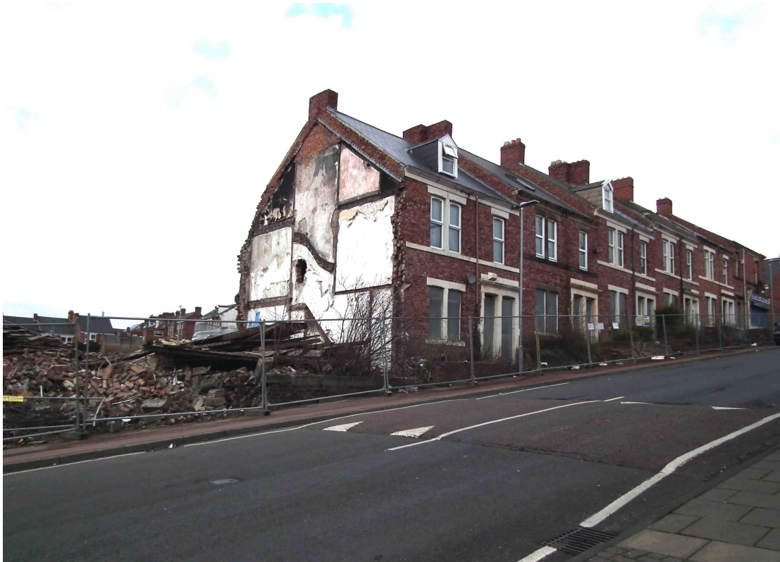
Dunsmuir Grove during demolition, March 2016. Source: author
