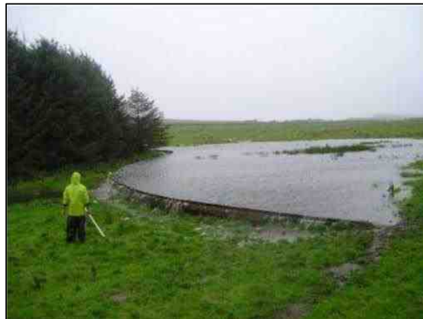
Figure 1.10 Examples of RAFs from Environment Agency (2011). A field bund temporarily storing overland flow during a storm event (top), a large woody debris dam (middle) and an offline storage pond constructed with a timber barrier (bottom).
