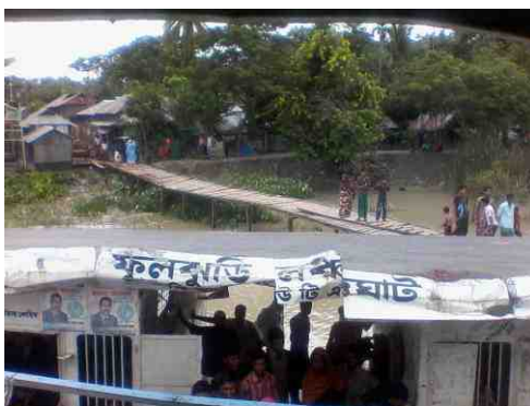
Damage in Cyclone Sidr in 2007, still unrepaired
