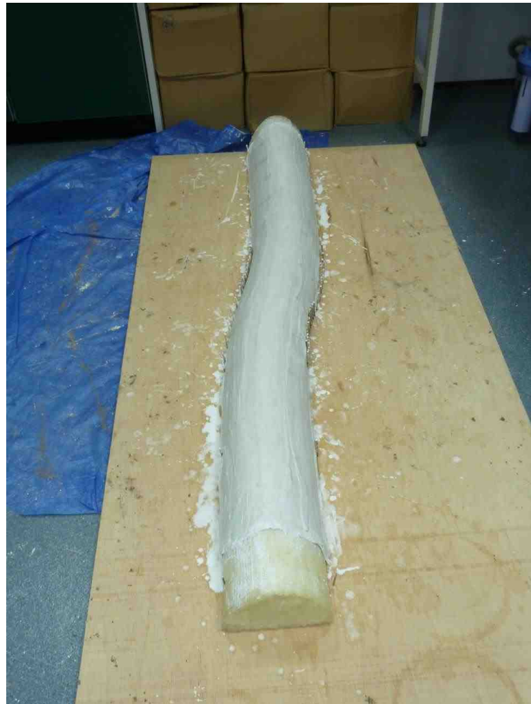
Figure 3.8: Manufacturing a channel bend. Here, the ModRoc layers have been applied to the foam mould, which is pinned for a curve of R_c = 0.7 m and \theta = 20^\circ
