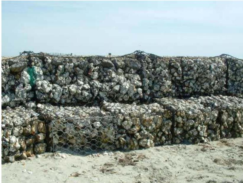
**Figure(6.7): Artificial Recharge using gabions**
