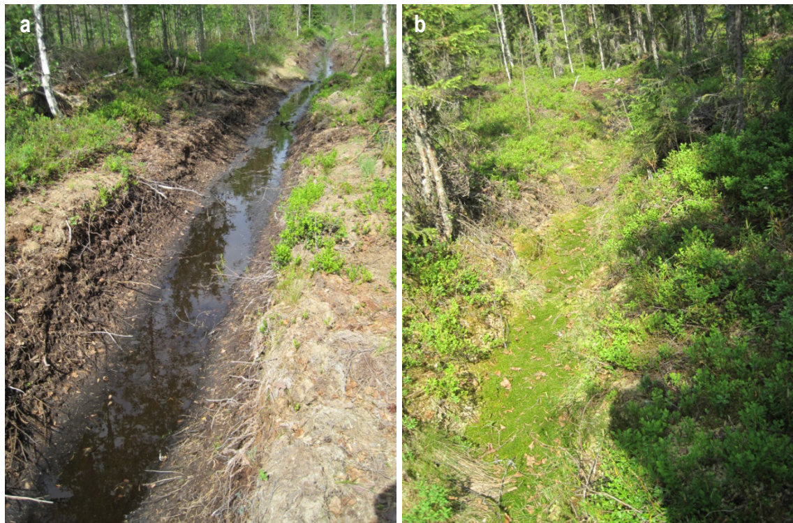
Figure 7 Example of maintained (a) and unmaintained (b) ditch in the Koivupuro nested catchment in Eastern Finland. (Pictures Kersti Hahti)
