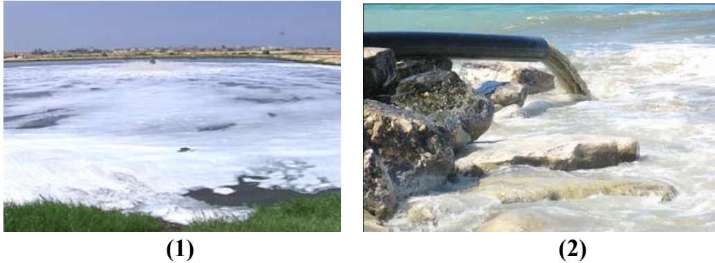
Figure (9): Wastewater problems (1): A sewage lagoon next to a sewage pumping station in Beit Lahia (2): Discharge of untreated wastewater into the sea from the existing Rafah Wastewater Treatment Plant, March 2009
