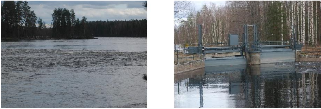
Figure 29. Kalkkinen natural cascade (left) and the regulation weir in Kalkkinen (right).
