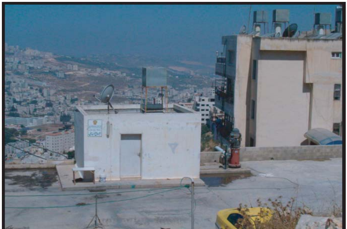
Northern Pumping Station and Reservoir
