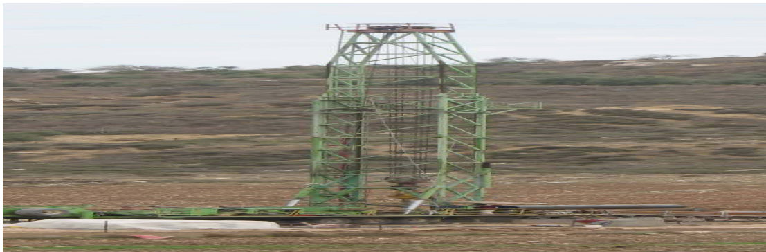
Figure 18. Sabastia Well during construction
