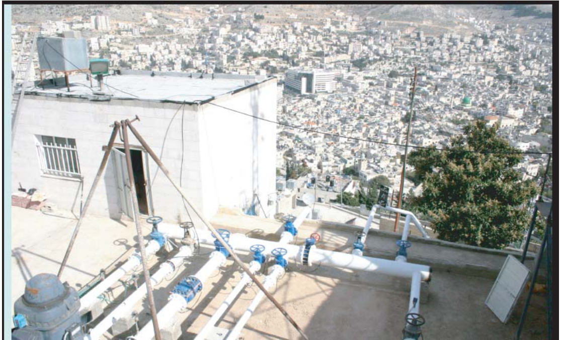
Southern Pumping Station and Reservoir
