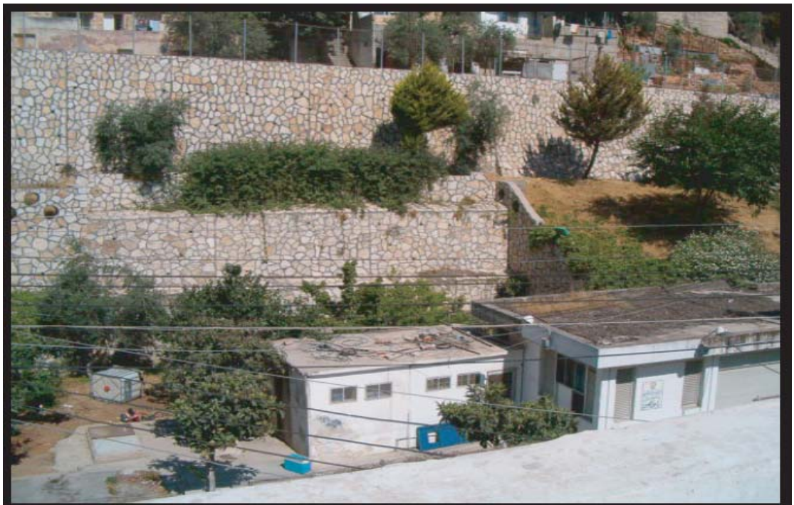
Ras Elein Pumping Station and Reservoir
