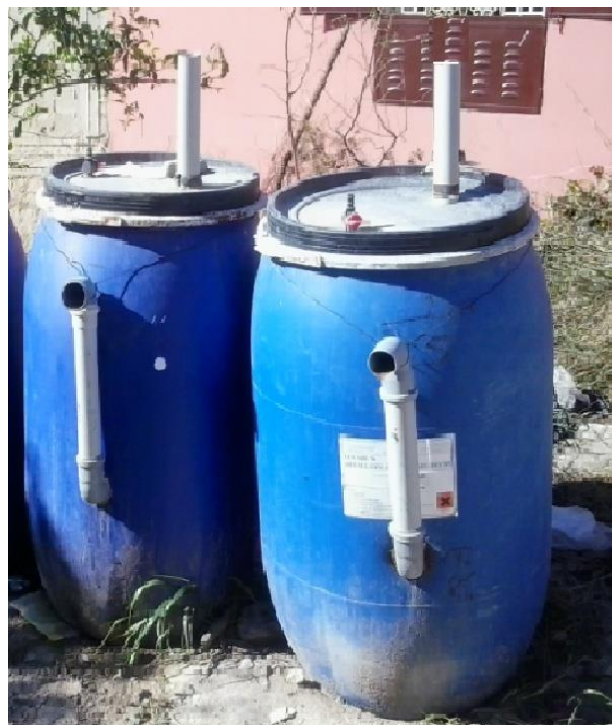
Figure 3.2: a photo of two typical biogas units
