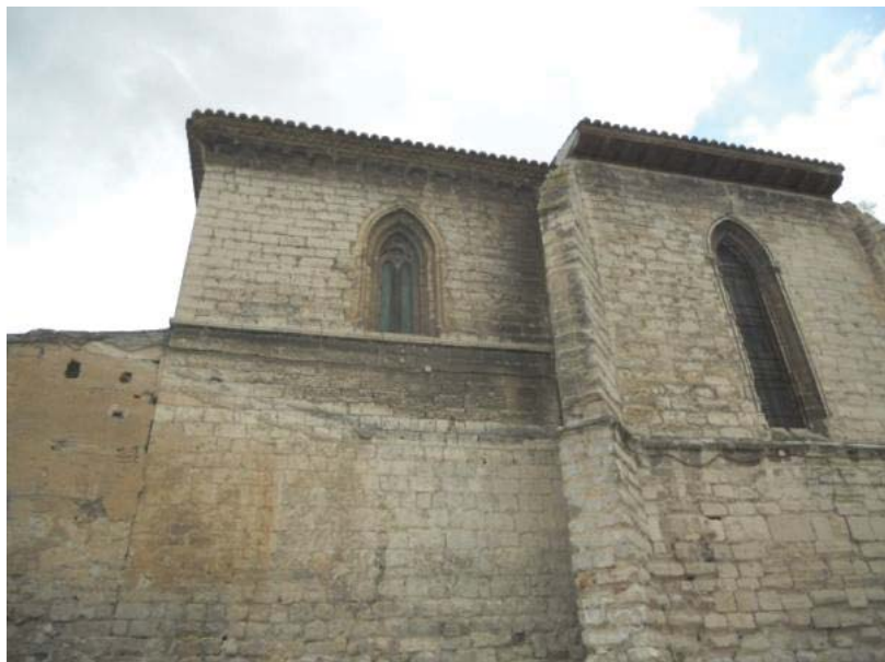
Figure 2.3. Thirteenth-century exterior walls of Santa María la Mayor, Valladolid. Photo by James E. Dory-Garduño, © 2011-13.
