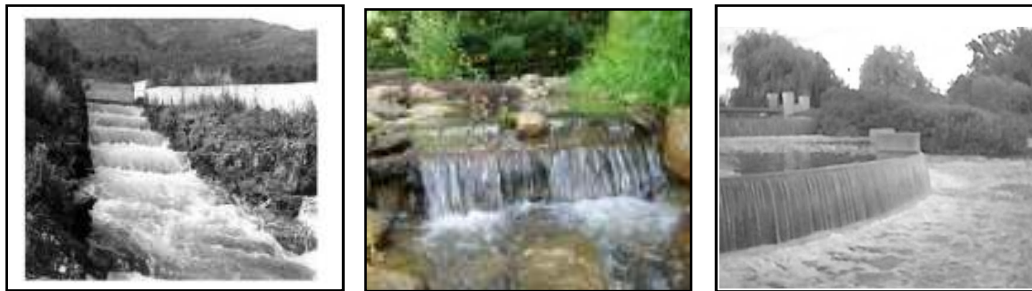
(a) (b) (c) Figure (5.6): Typical in Stream Aeration Techniques: (a) Ladders [49], (b) Waterfalls, (c) Side-Stream Aeration [9].
