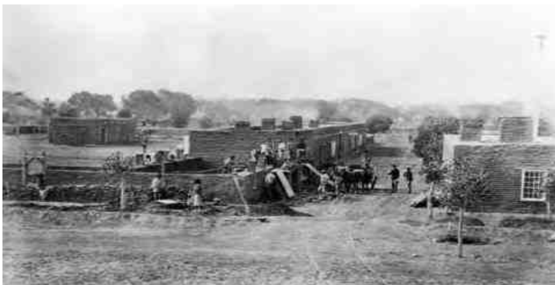
Figure 9. It appears that Natives are participating in Fort Sumner's construction while soldiers stand guard. "Fort Sumner Construction," Center for Southwest Research, University Libraries, University of New Mexico, accessed July 26, econtent.unm.edu/cdm/singleitem/collection/Bunting/id/21/rec/1282016
