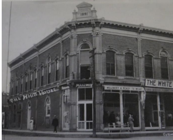
Catron Building, northwest corner, facing Santa Fe Plaza, New Mexico, c. 1915. Law Office of Thomas B. Catron, III, Santa Fe.
