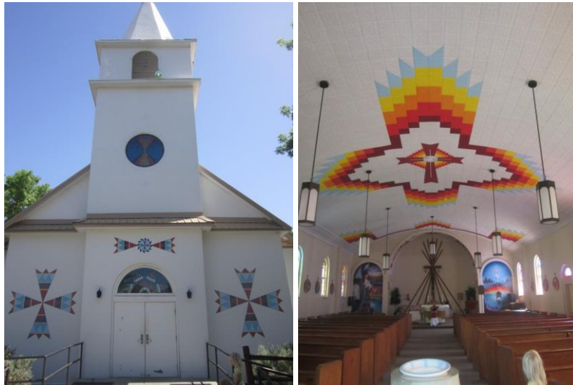
Figure 9. Exterior and interior of St. Stephens Church, 2013. Photograph courtesy author.
