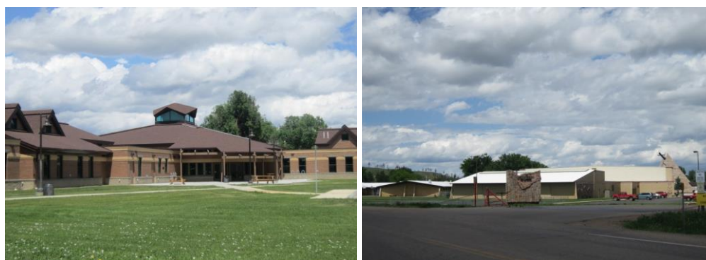
Figure 14. Right , newly-constructed dorm dedicated on 23 September 2011. Left , entrance to St. Labre Indian School complex, 2013. Photograph courtesy author.
