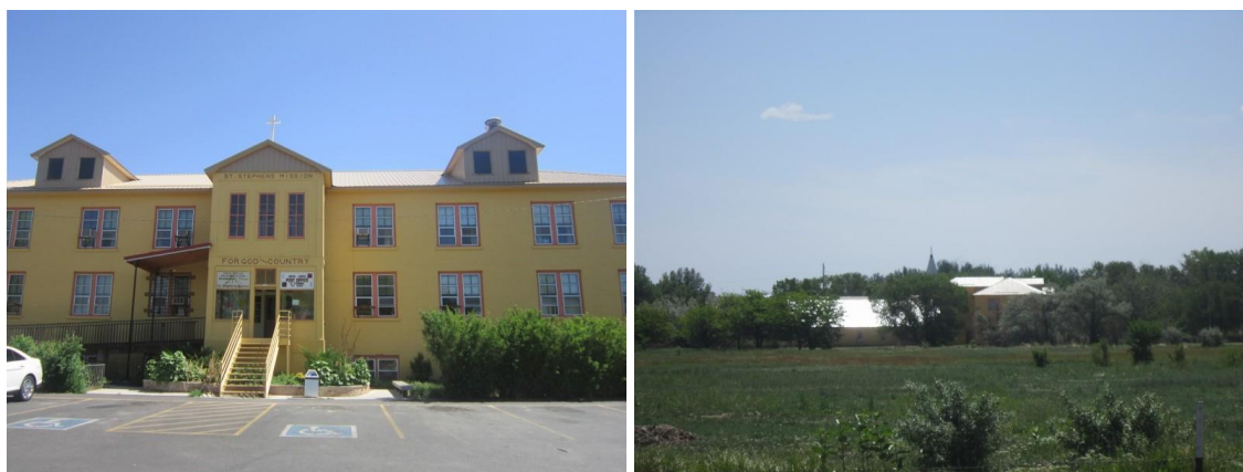
Figure 7. Left , the old boy's dormitory and classrooms built in 1928 now serves as a museum, gift shop, post office, and community center in St. Stephens, Wyoming. Right , view of the mission complex, 2013. Photograph courtesy author.
