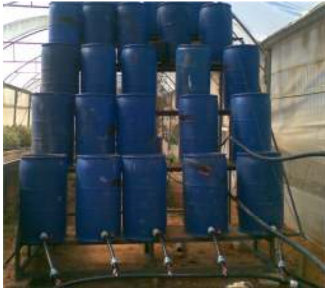
Figure (3-3):(4-stages)VF sub-surface constructed wetland An-Najah National University 2010.
