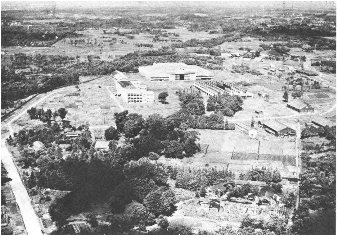
Aerial view of ICU campus in late 1940s. Note the farming fields still present.
