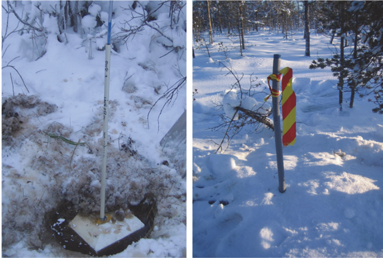
Fig. 5. Ground frost pipe installation in (left) the Pehkeensuo wetland and (right) ground frost pipe with protection tube in the Kapustaneva wetland (photos by H. Postila).
