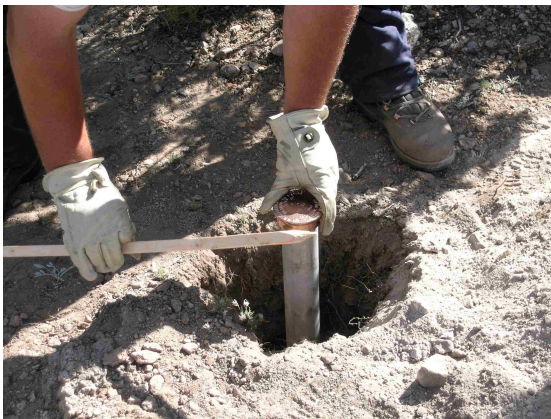
Figure 35. Setting the newly-surveyed corner brass cap.
