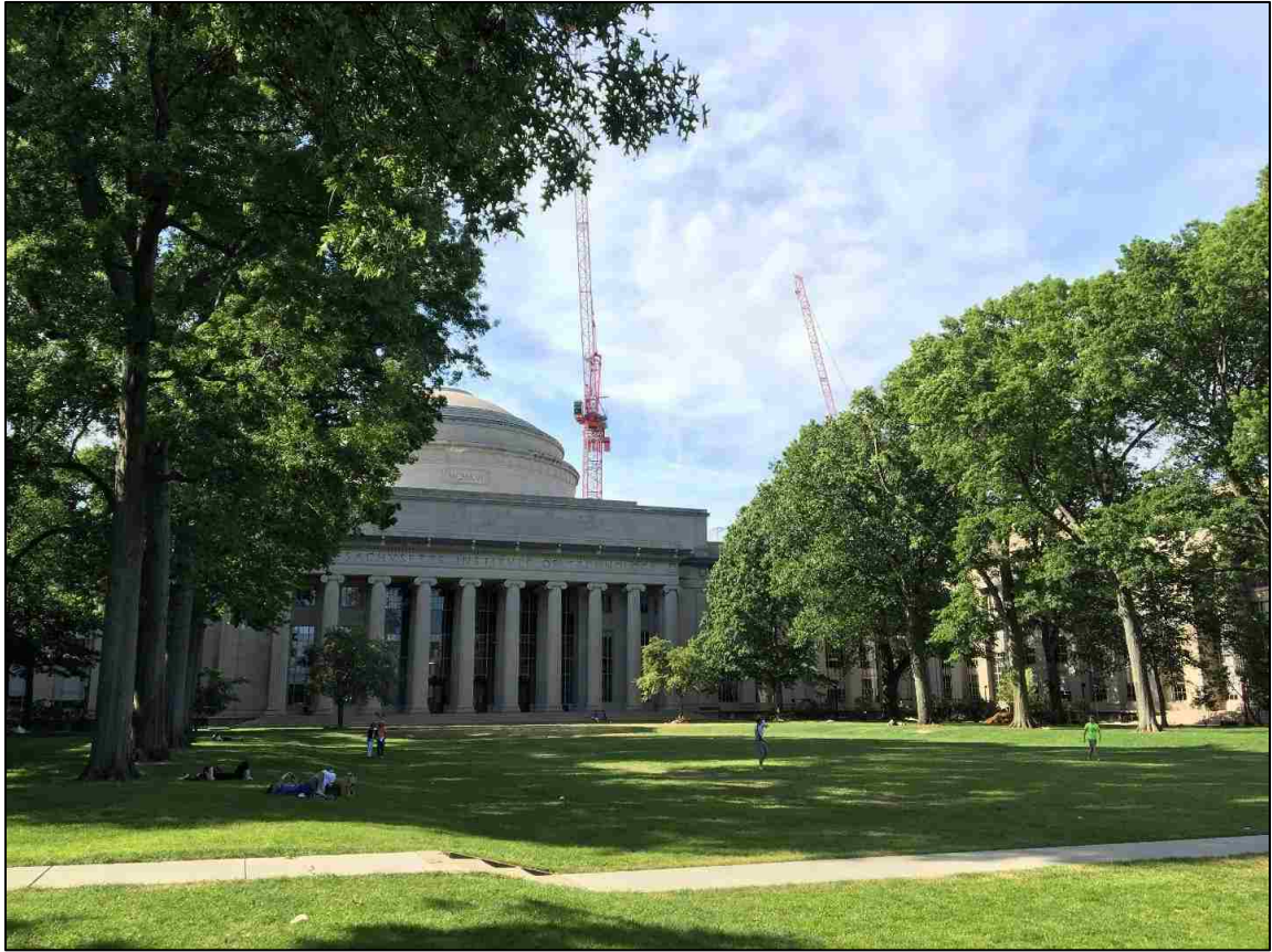
Figure 2. Construction at the Massachusetts Institute of Technology
