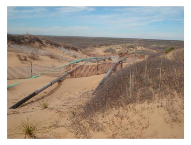
Figure 1: Pipelines Exposed by Blowout . Blowout on right of way located within the Mescalero sand sheet. Photo: Knutt Peterson
