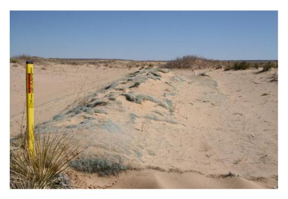
Figure 10: One year old geotextile repair, placed over sand mounded on top of exposed pipeline. Geotextile is already being torn away from repair. Photo: Knutt Peterson
