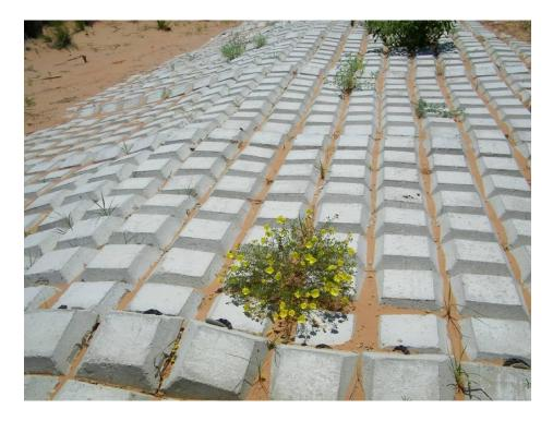
Figure 8: Articulating concrete mat at one of Submar's testing sites in Southeast New Mexico. Photo courtesy of Submar.
