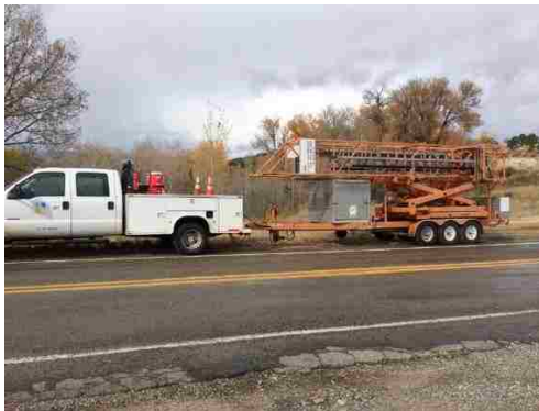
Figure 96. Mobile Scaffold from NMDOT District 4
