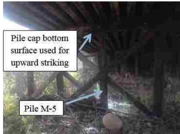
Figure 105. Photo of Pile M-5 and the Pile Cap
