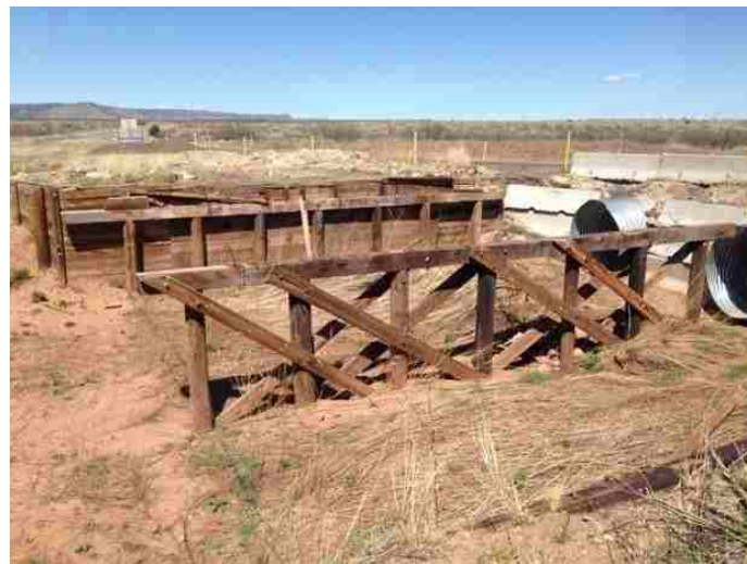
Figure 124. Photo of the Partially Dismantled Bridge near Route 419
