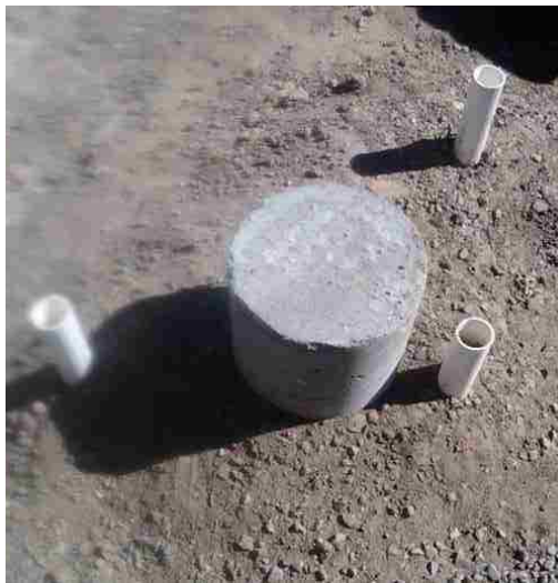
Figure 184. Layout of the Concrete Pier and Boreholes
