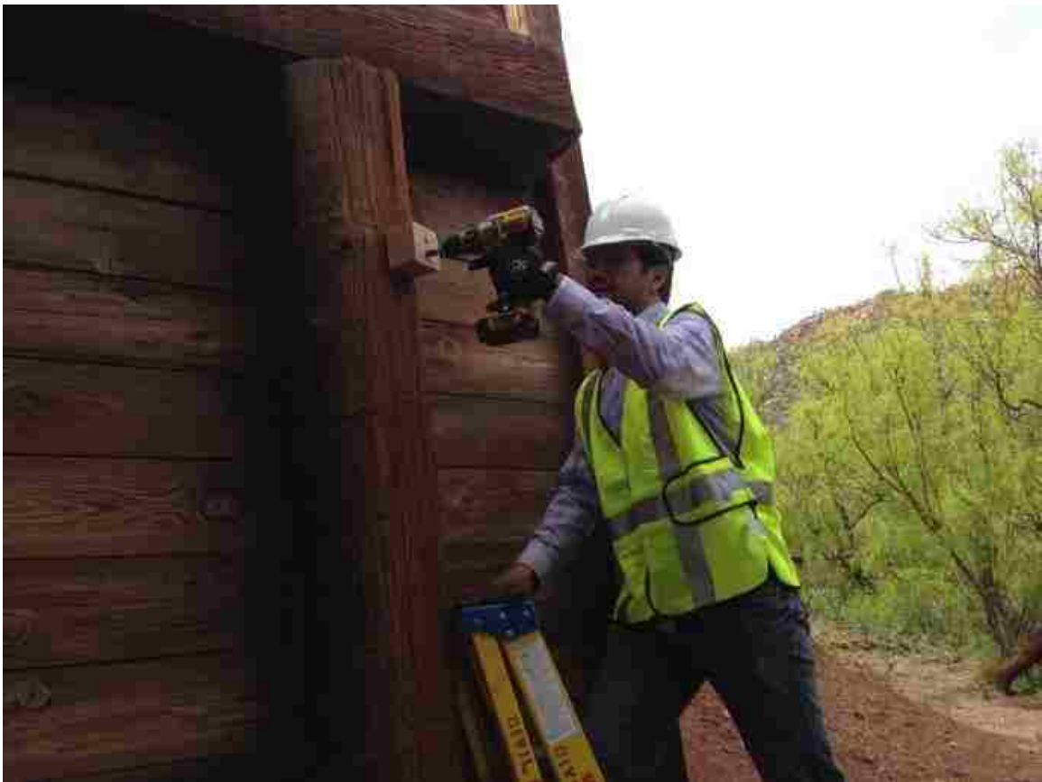
Figure 25. Attachment of a Wooden Striking Block onto the Test Pile
