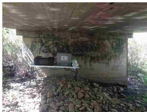
Figure 132. Side View of One of the Piers
