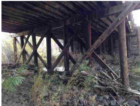
Figure 94. Photo of Bridge No. 1190 during the Second Visit
