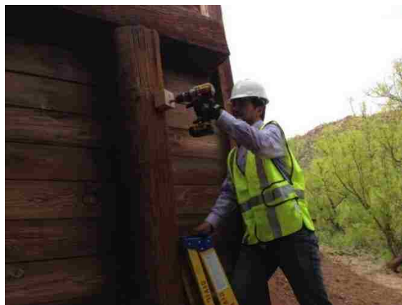
Figure A13. Attaching the Striking Block on the Test Pile
