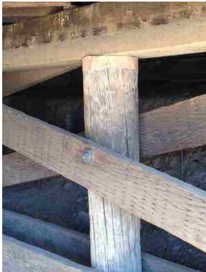
Figure A15. Diagonals and a Bolt
