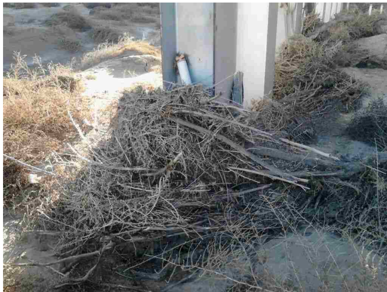
Figure 147. Destroyed Pipe (B-06)
