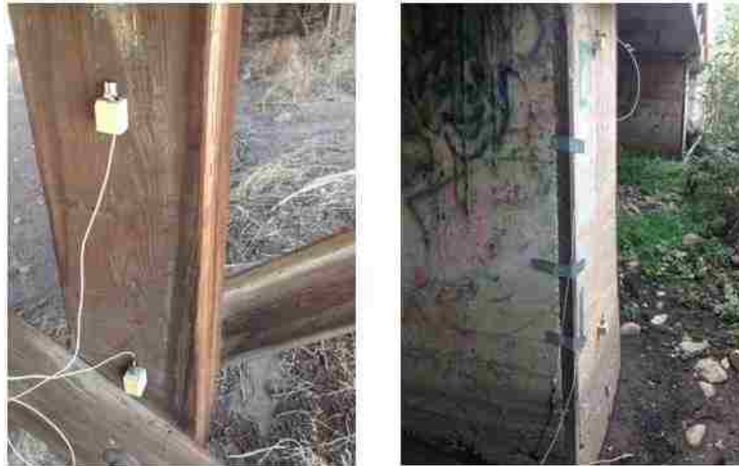
Figure A19. Two Accelerometers Mounted on the Side of the Substructure
