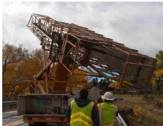
Figure 97. Preparing the Mobile Scaffold
