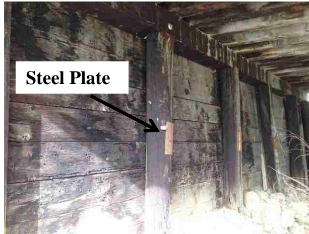
Figure 103. A Steel Plate Attached to Pile 10
