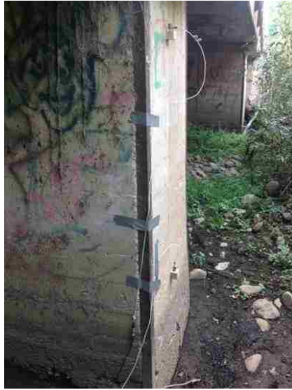
Figure 134. Attached Accelerometers on the Pier Side
