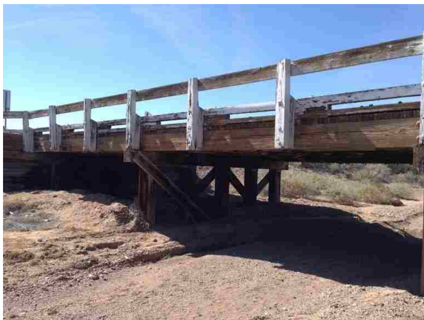
Figure 116. Street View of Bridge No. 1676
