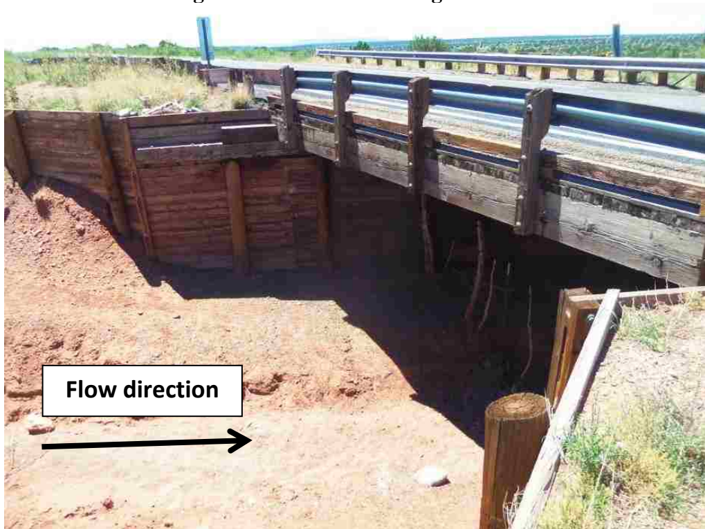
Figure 61. Street View of Bridge No. 6922
