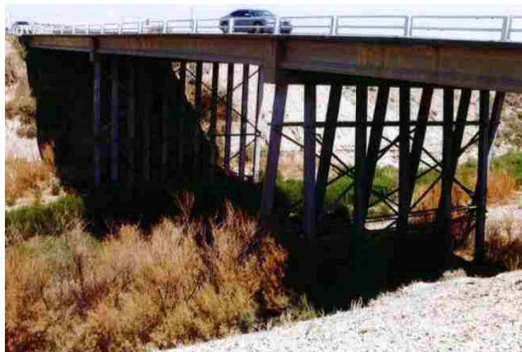
Figure 127. Street View of Bridge No. 7480
