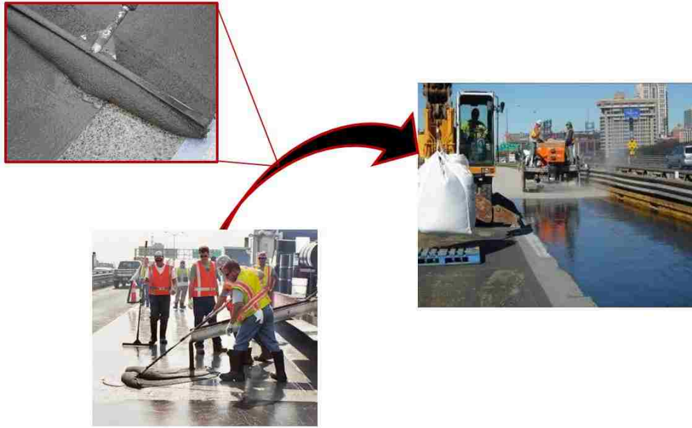
Figure 2.6: PC overlays in-situ courtesy of Transpo Inc.
