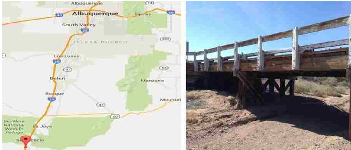
Figure 3-16: Location and Street View of Bridge #1676
