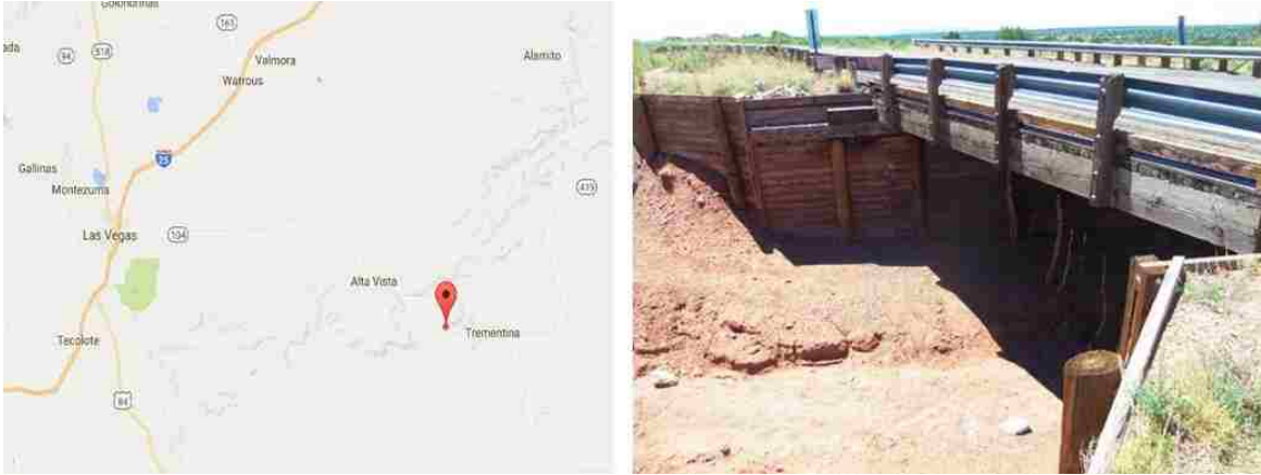
Figure 3-18: Location and Street View of Bridge #6922
