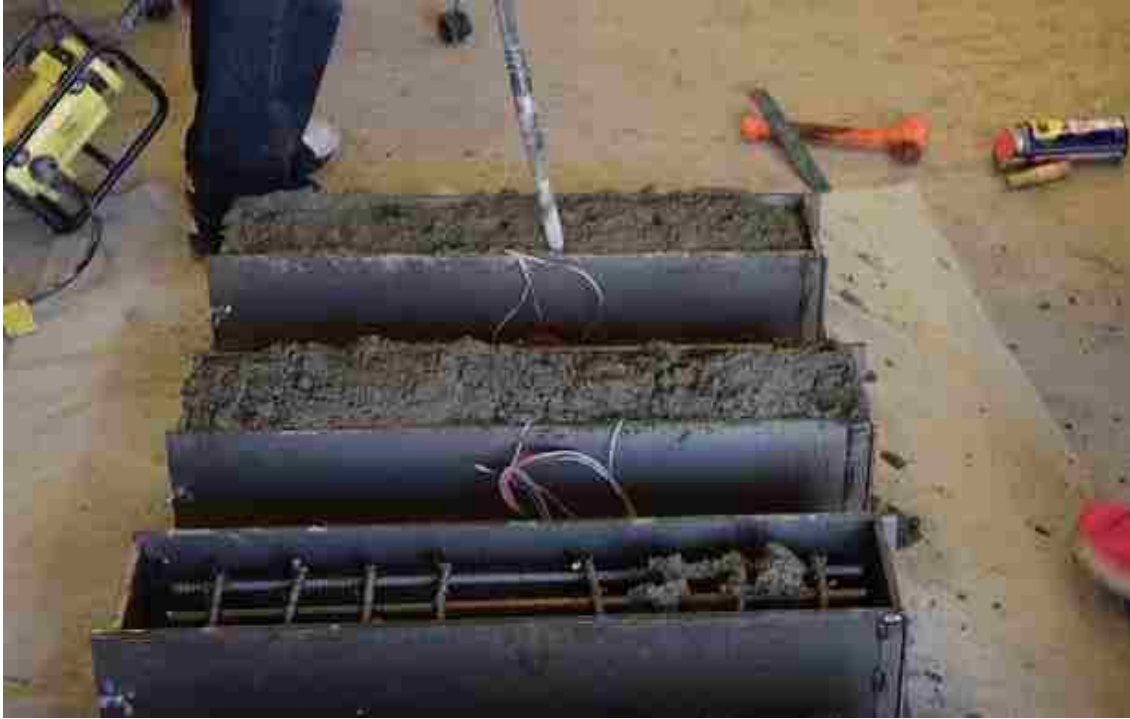
Figure 3.6: Concrete compaction using vibrator
