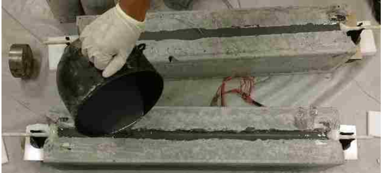
Figure 3.9: NSM groove being filled with epoxy
