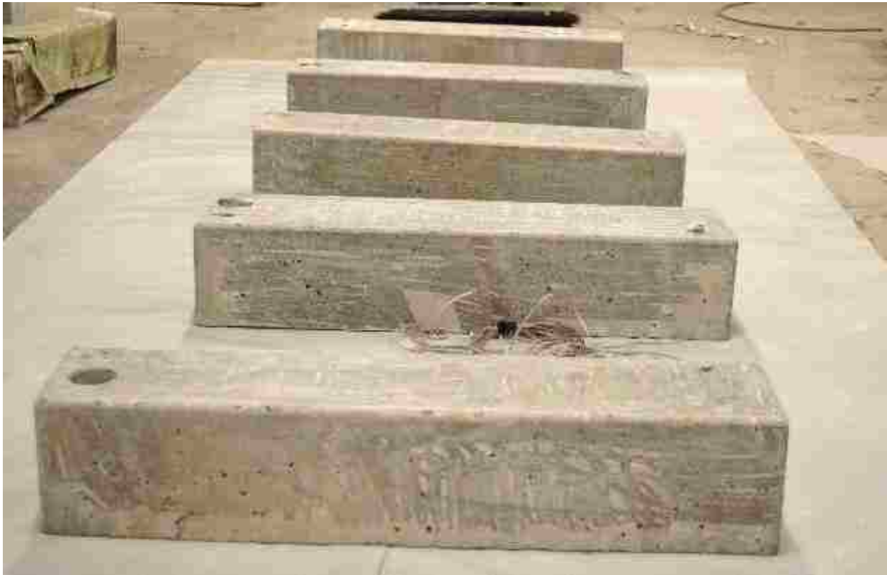
Figure 3.10: Grinded RC beams ready for FRP wrapping
