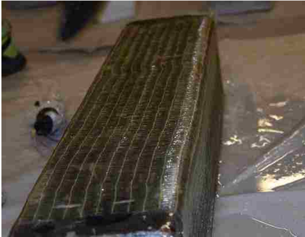
Figure 3.15: Beam after U-wrapping with GFRP fabric for shear strengthening
