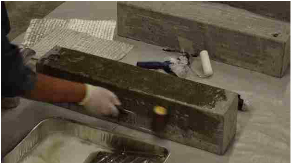
Figure 3.13: Prime coat with adhesive before GFRP wet-layup
