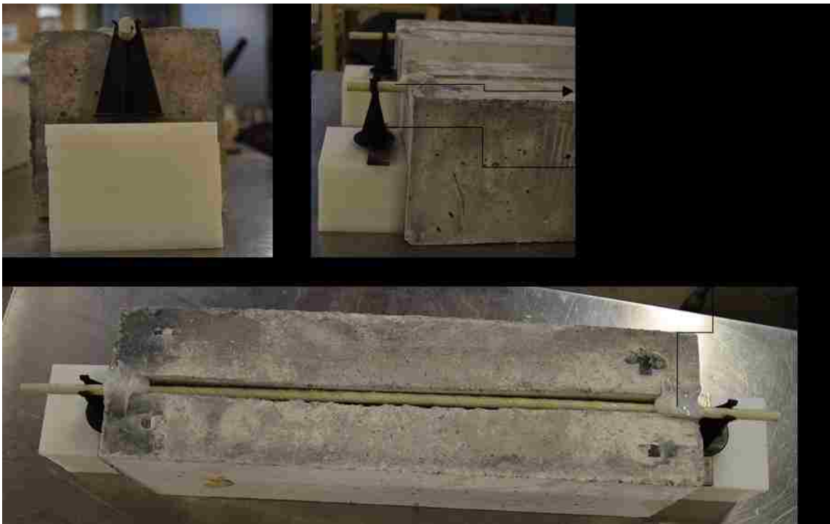
Figure 3.8: NSM groove with GFRP bar before pouring the adhesive
