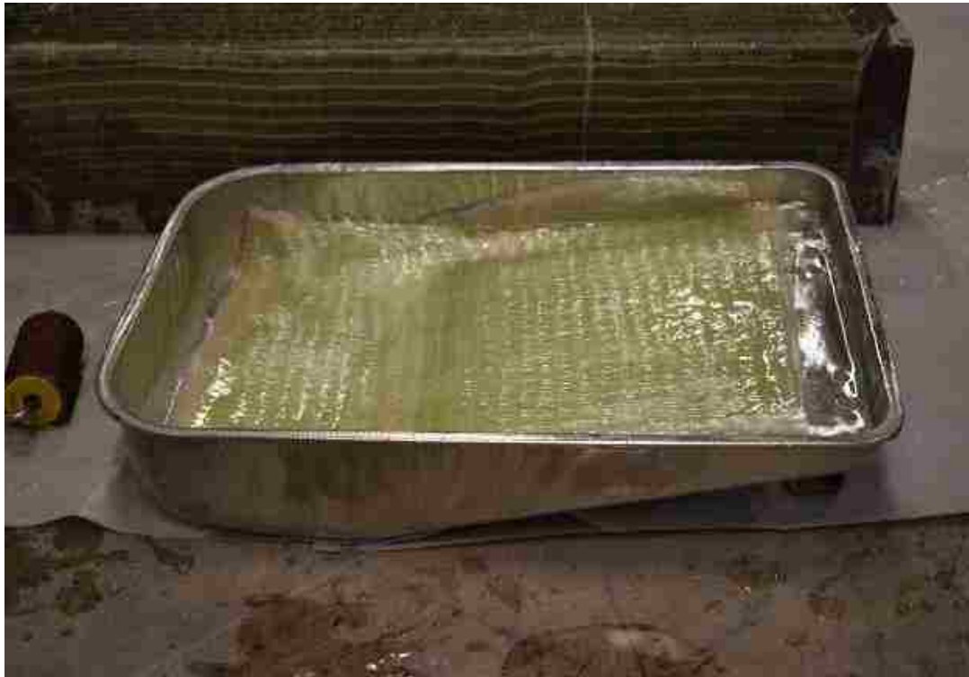
Figure 3.14: GFRP fabric saturated in adhesive
