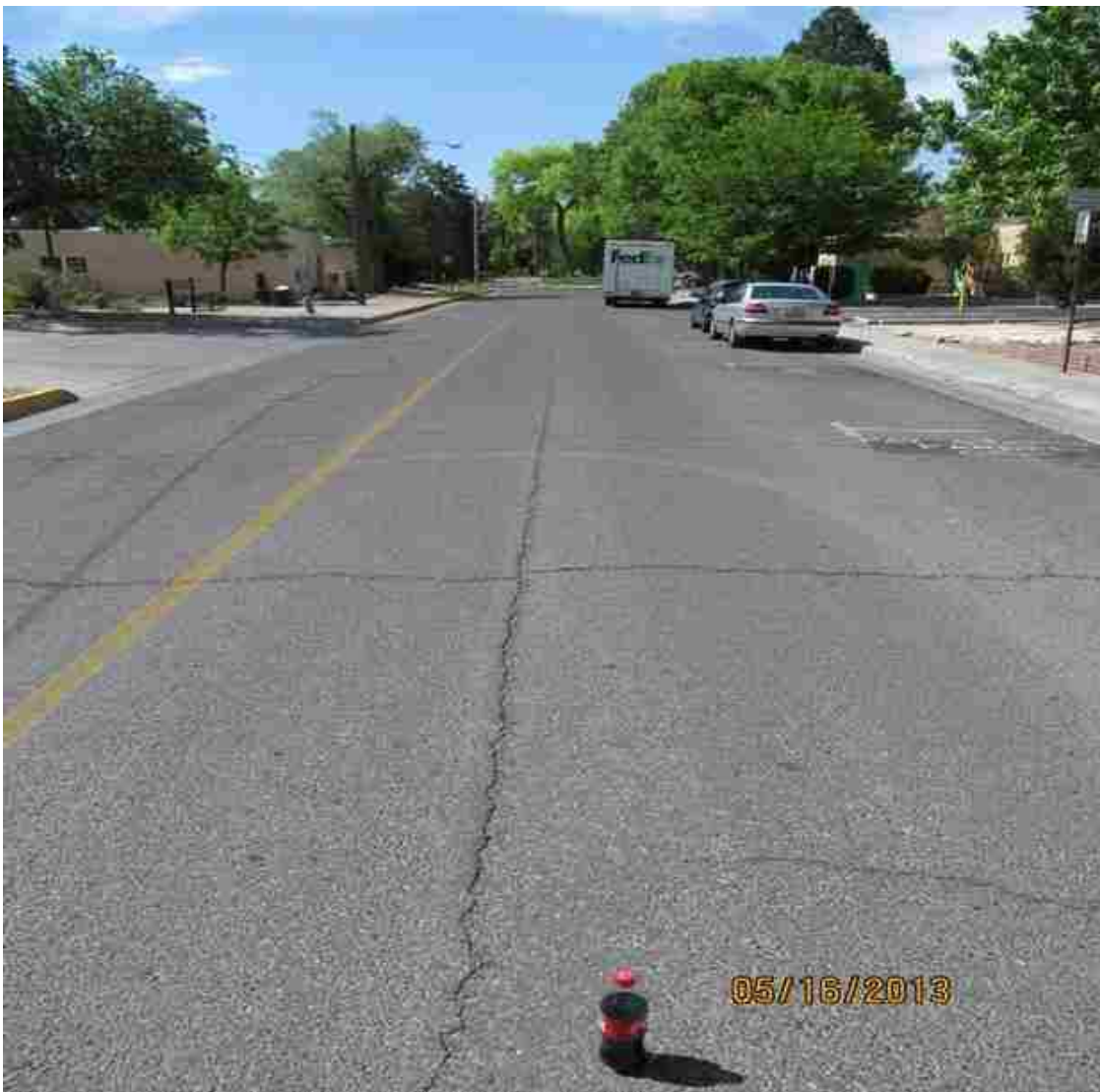
Figure 7. Longitudinal cracking
