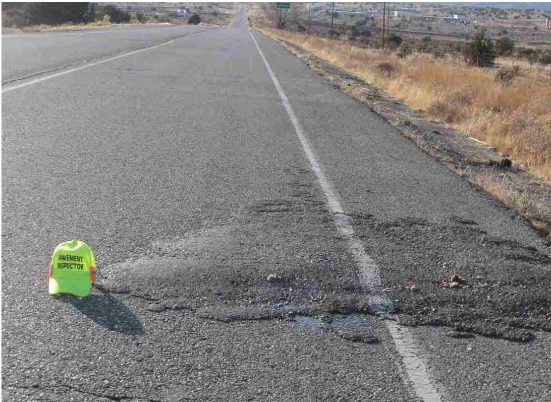
Figure 6. Pavement patching
