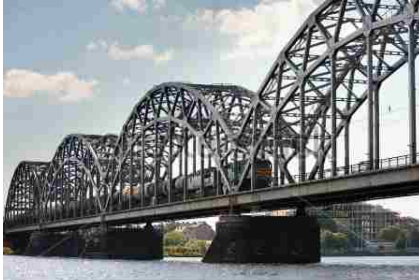
Fig. 1.4. Railroad bridge under service load.
