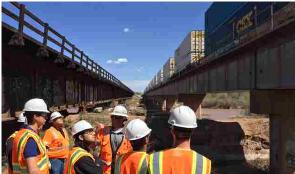
Fig. 1.3. Railroad bridge visual inspection.
