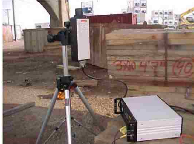
Fig. 2.4. Measurement of a railroad bridge vibration using a LDV (Nassif et al. 2005).
