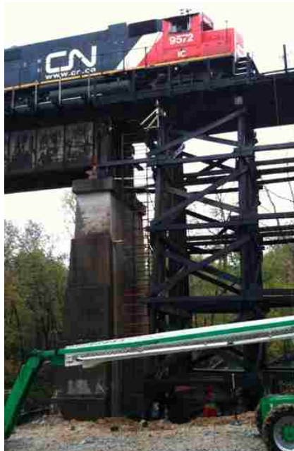
Fig. 2.2. Scaffolding to provide fixed reference point for displacement measurement of a railroad bridge (Moreu et al. 2015).
